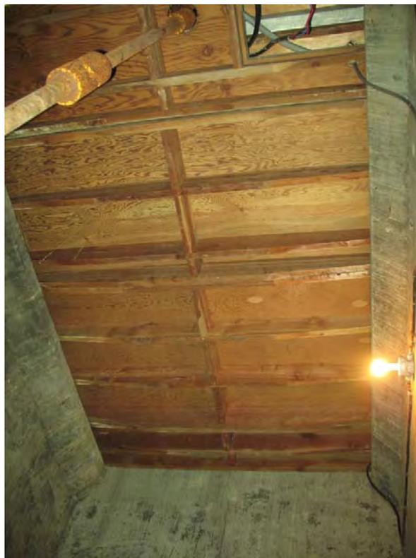
**Figure 6 - VC4 - Bottom of Existing Wood Floor**
