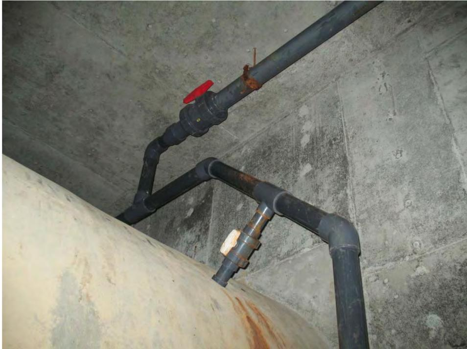
**Figure 19 - Chlorine Contact Chamber - Existing Injector Piping at Pipe**
