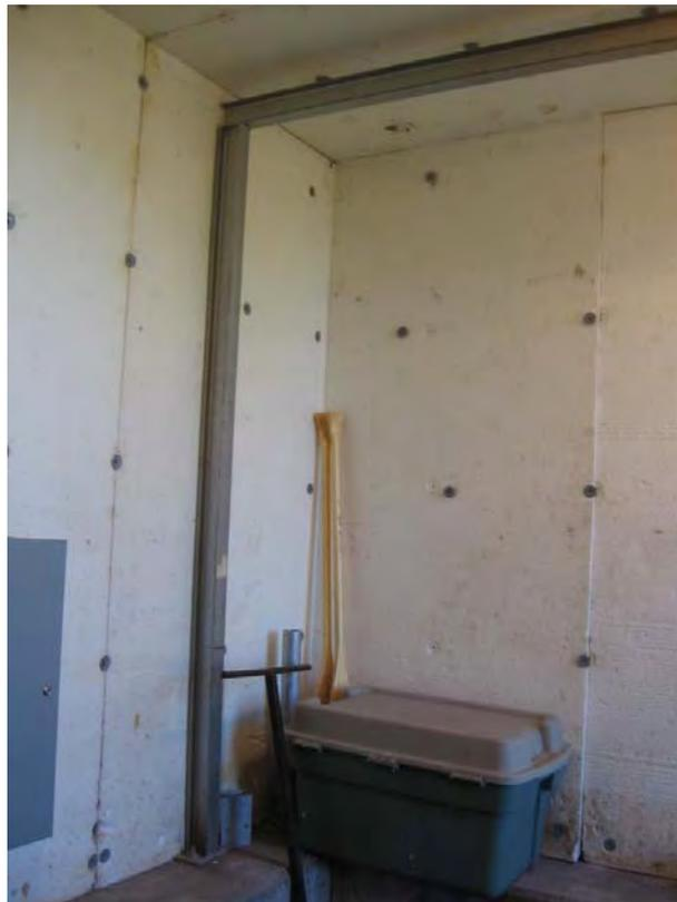
**Figure 16 - Cell 1 Dewatering Pump Station - Lifting Frame and Insulation**
