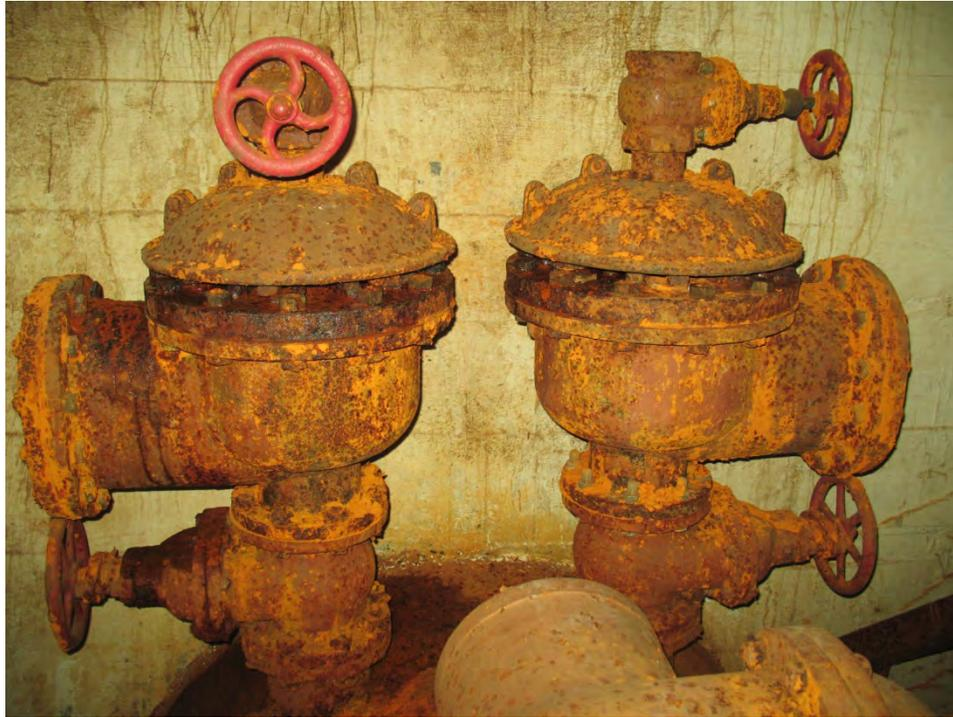
**Figure 11 - DAV1 - Existing Air Release Valve Assemblies**
