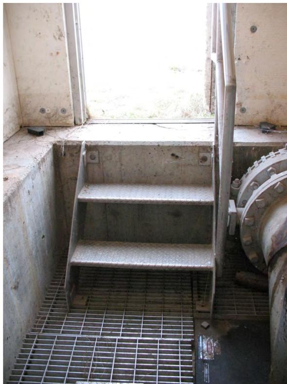
**Figure 14 - Cell 1 Dewatering Pump Station – Existing Stairs**
