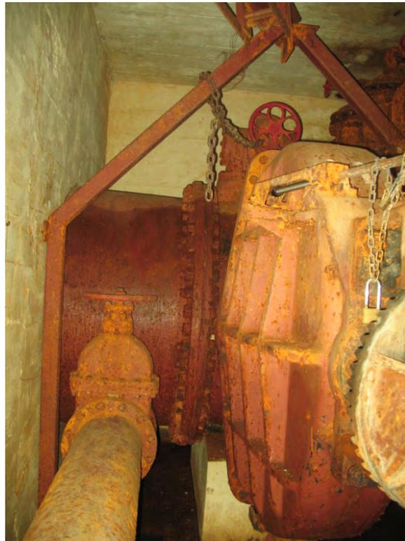
**Figure 12 - DAV1 - Existing 300 mm Gate Valve and Drain Piping**
