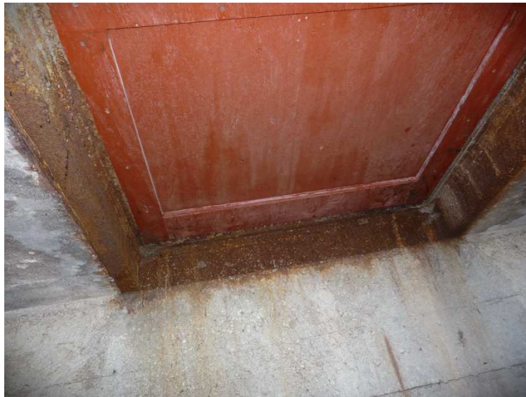
Figure 2-3 : Comminutor Chamber Access Hatch Surround
