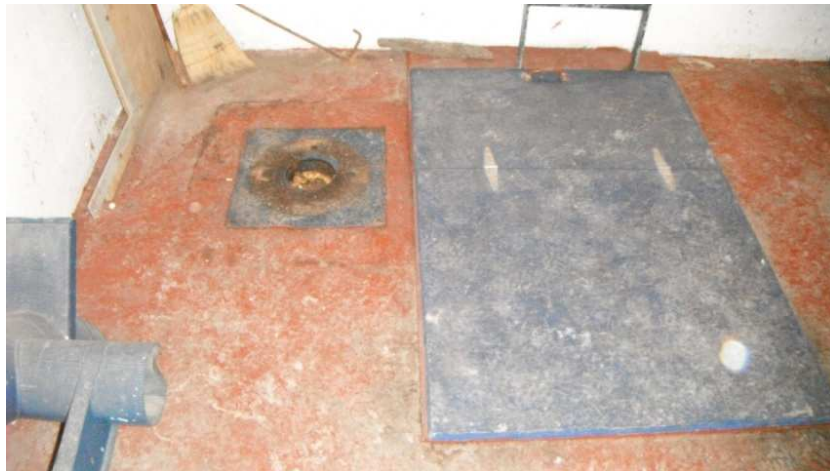
Figure 2-2 : Comminutor Motor Mount and Chamber Access Hatch
