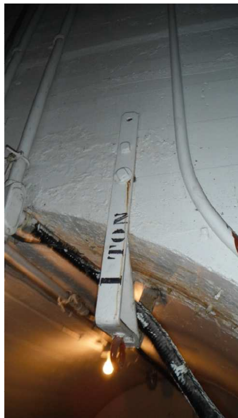
Figure 2-5: Motor Room Lifting Bracket
