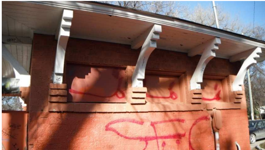
Figure 2-8 : Plywood Window Covers
