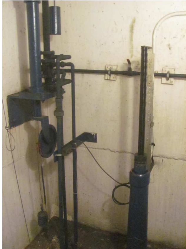
Figure 3-2 : Hydraulic Valve Actuator
