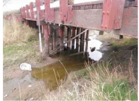
Drain site with bridge.
