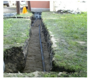
Typical trenching seen with permanent installation.
