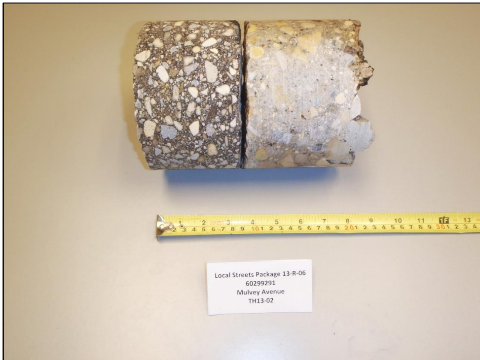
Photograph 2. Mulvey Avenue – TH13-02
