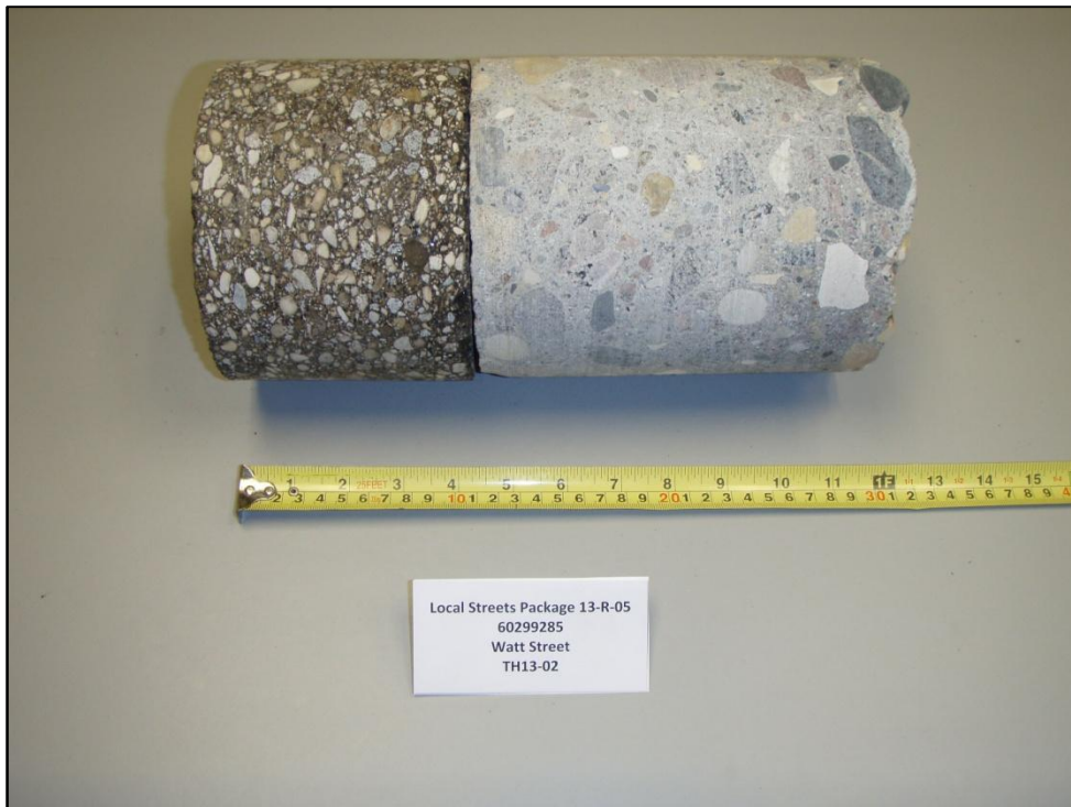
Photograph 2. Watt Street – TH13-02
