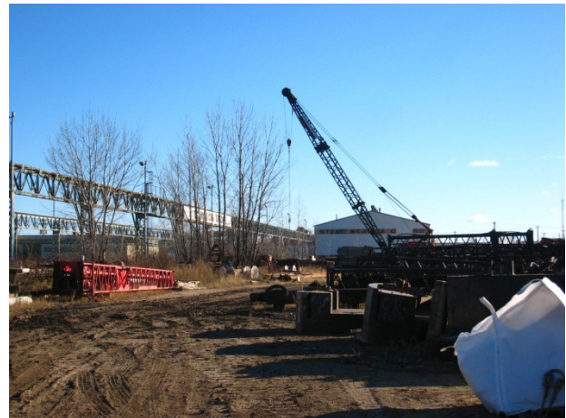
Photograph 15 ↑ View of landfilling area facing east
