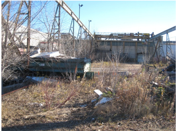
Photograph 17 ↑ View of BH10-57 facing east
