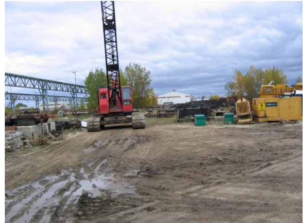
Photograph 13 ↑ View of landfilling area facing east
