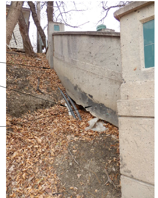
5 EXISTING PHOTO - EXPOSED CONDUITS Scale: 1:200
