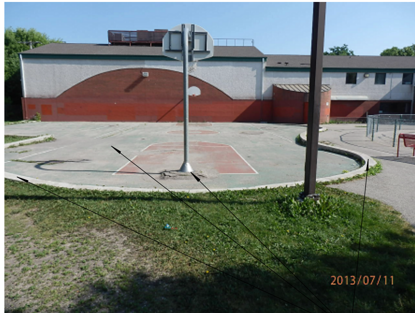
PHOTO "4": EXISTING ASPHALT PAVING AND CONCRETE CURBS TO BE REMOVED. BASKETBALL POST AND FOOTING TO BE REMOVED.
