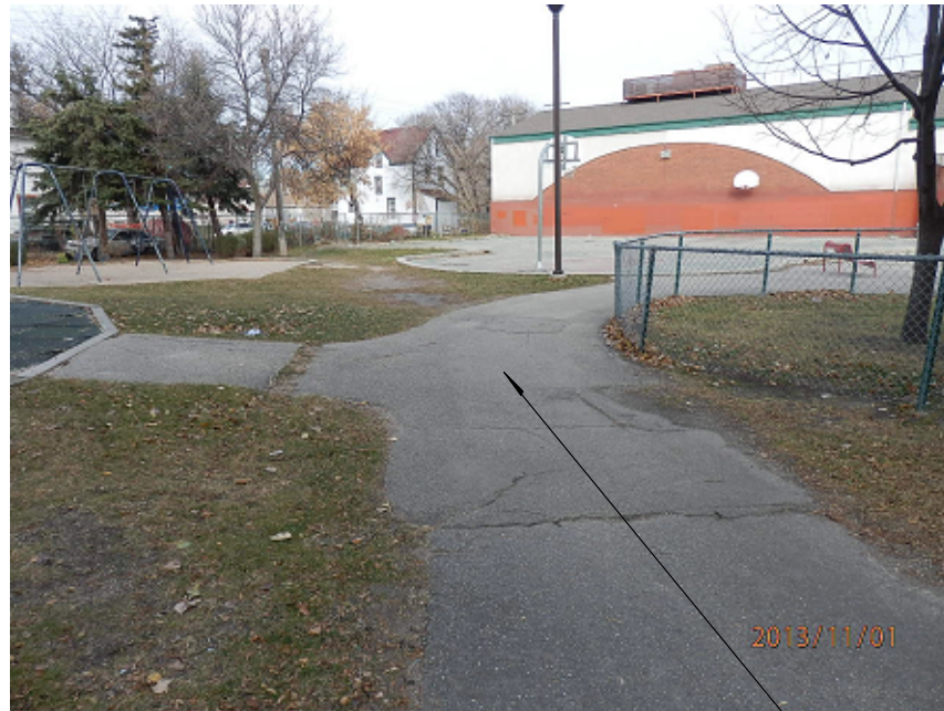
PHOTO "14": ASPHALT WALKWAY AND GRASS TO BE PROTECTED.
