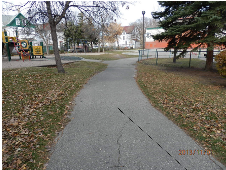
PHOTO "13": ASPHALT WALKWAY AND GRASS TO BE PROTECTED.
