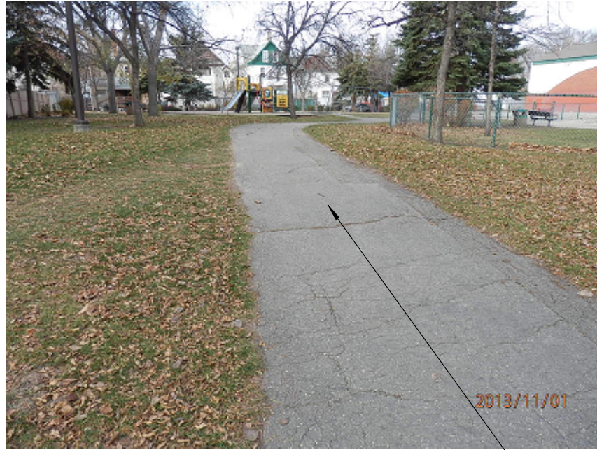
PHOTO "12": ASPHALT WALKWAY AND GRASS TO BE PROTECTED.
