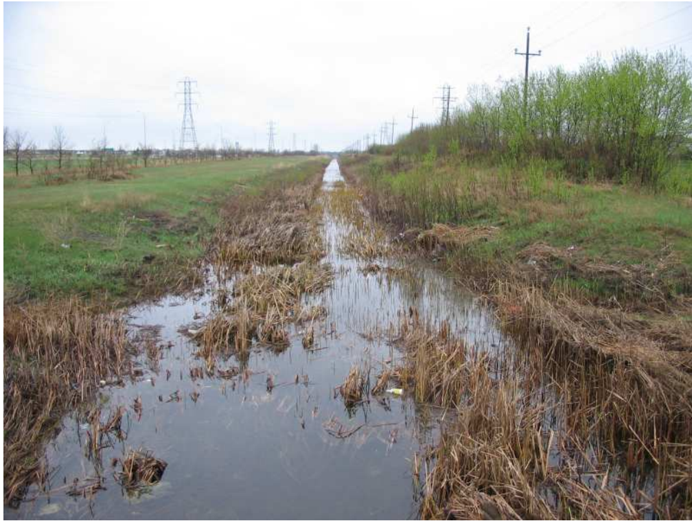
Photo No. 1 Navin Drain west of Lagimodiere Boulevard (May 2005)
