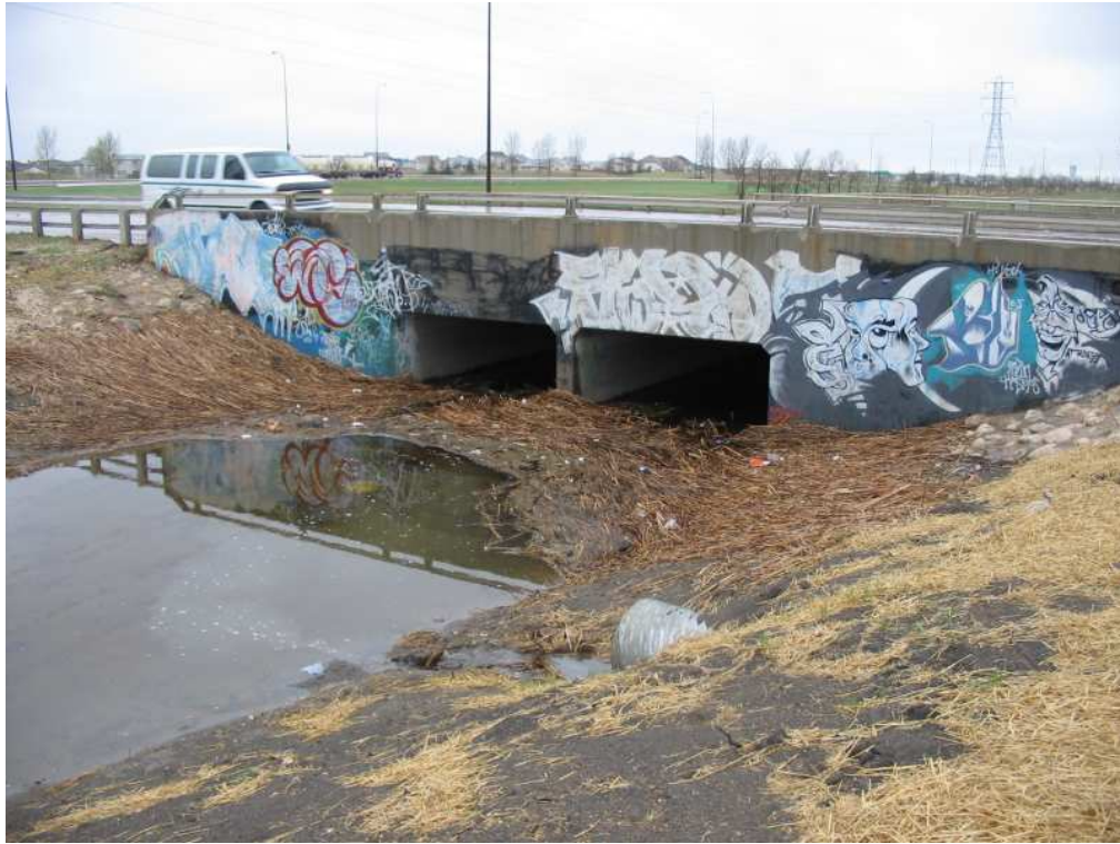
Photo No. 3 East side of Lagimodiere Boulevard Crossing (May 2005)
