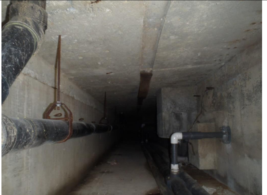
Photograph #3: Mechanical tunnel – outside wall on left.
