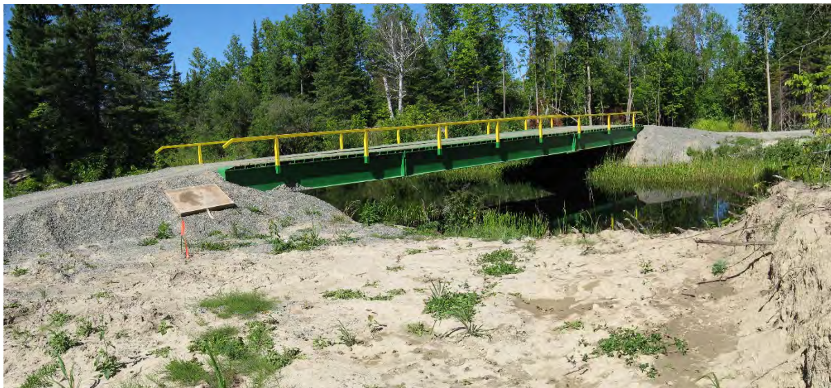
Figure 02 View North at Temporary Bridge
