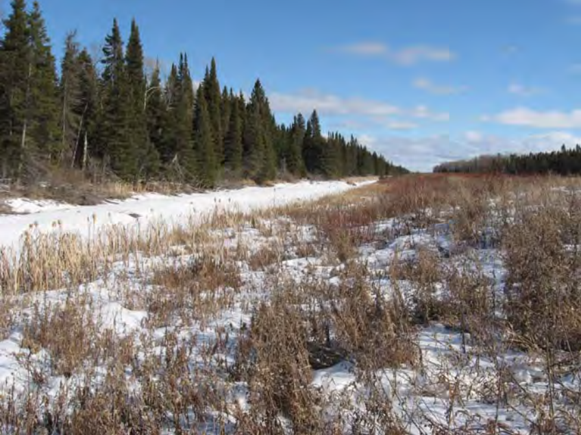
Mile 93 Shoal Lake Aqueduct - February 17, 2012
