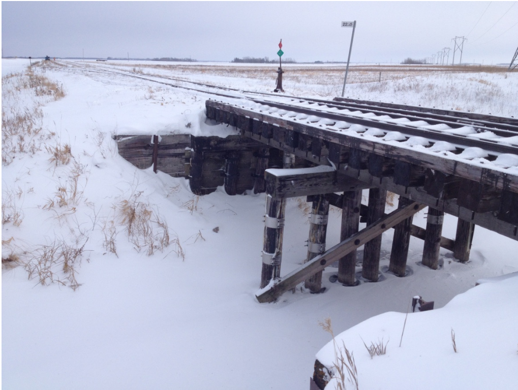
Photo 1: Existing Bridge Foundations, Looking Southeast.
