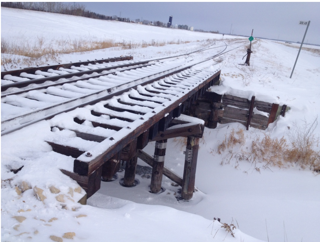
Photo 2: Existing Bridge Foundations, Looking North of east.
