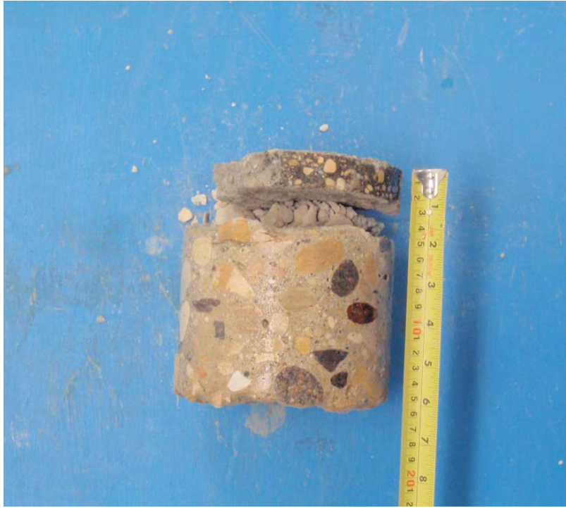
Core sample from Testhole TH03
