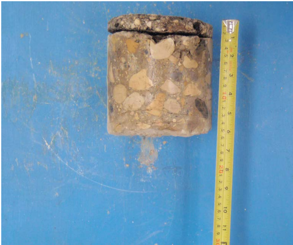
Core sample from Testhole TH06
