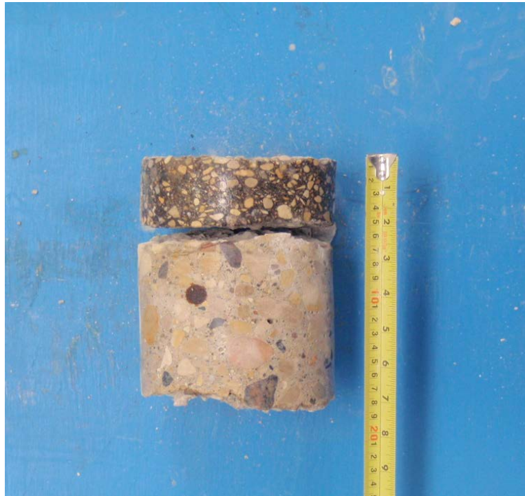
Core sample from Testhole TH01
