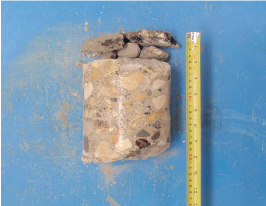
Core sample from Testhole TH01
