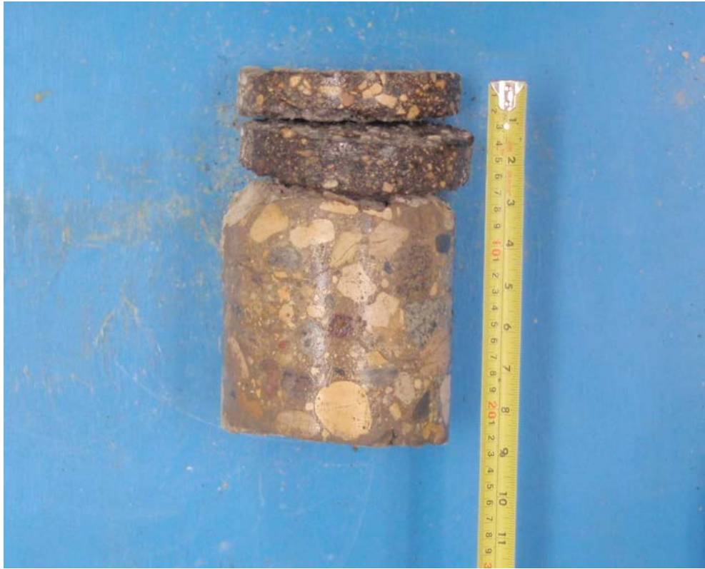
Core sample from Testhole TH05
