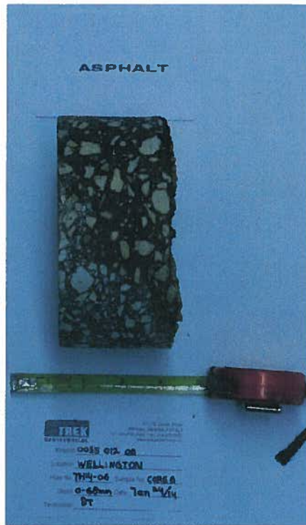
Photo 13: Asphalt Core Sample from Test Hole TH14-06
