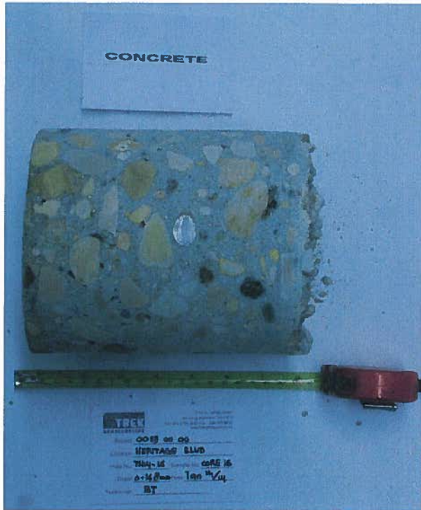
Photo 3: Asphalt and Concrete Core Sample from Test Hole TH14-16
