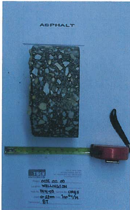
Photo 9: Asphalt Core Sample from Test Hole TH14-05
