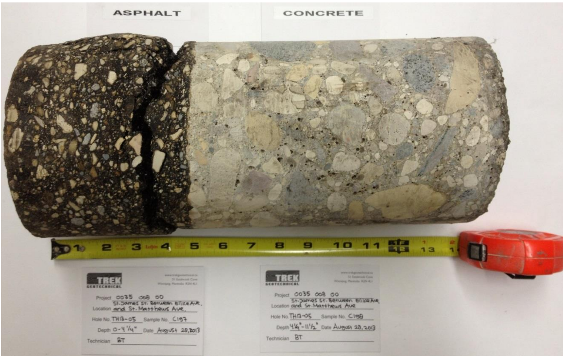
Photo 4: Asphalt and Concrete Core Sample from Test Hole TH13-05
