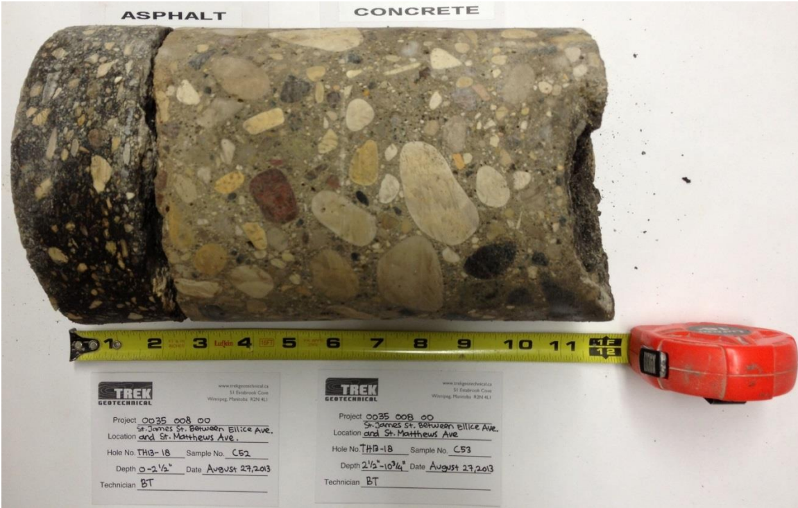
Photo 15: Asphalt and Concrete Core Sample from Test Hole TH13-18
