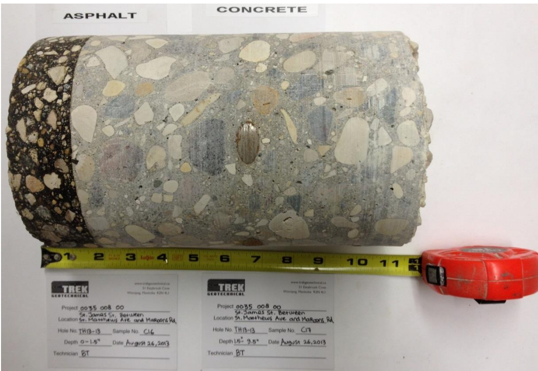
Photo 10: Asphalt and Concrete Core Sample from Test Hole TH13-13
