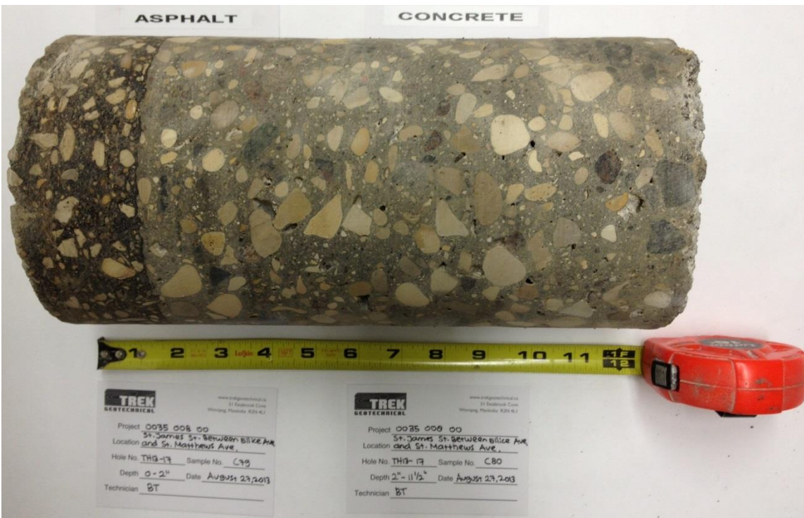
Photo 14: Asphalt and Concrete Core Sample from Test Hole TH13-17
