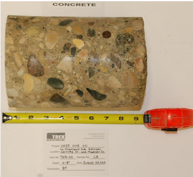
Photo 2: Concrete Core Sample from Test Hole TH13-02
