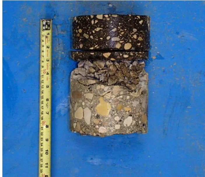
Core sample from Testhole TH2
