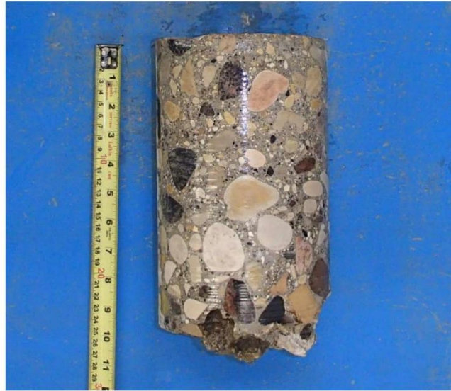
Core sample from Testhole TH1
