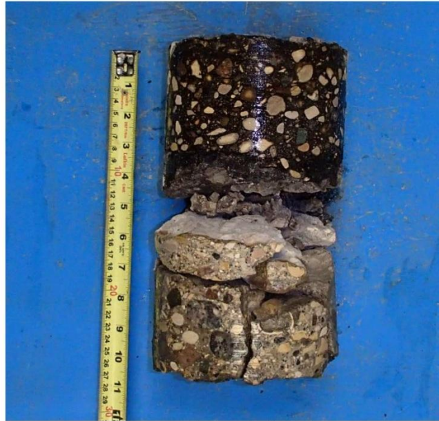
Core sample from Testhole TH3
