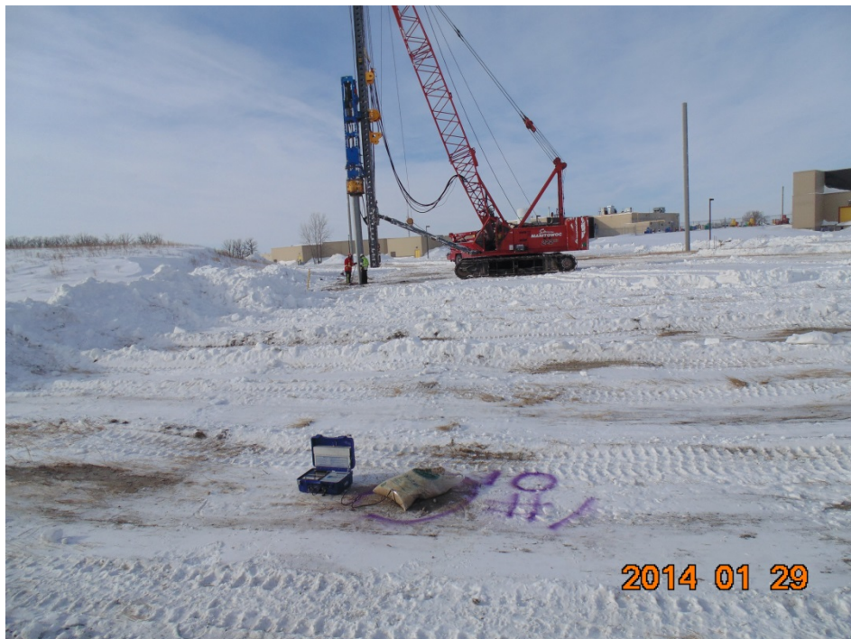
Photo 2 – Pile #1, showing monitor M1
