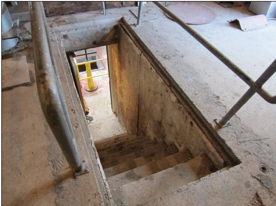
Figure 50 – Main floor opening / stairwell to first sublevel.
