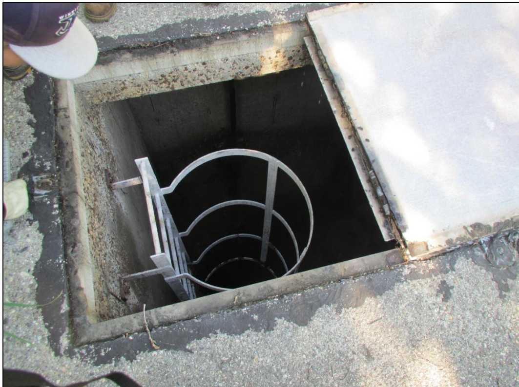
Figure 14 – Chamber access / interior.
