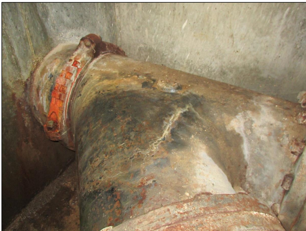
Figure 40 – Chamber interior, upstream direction.
