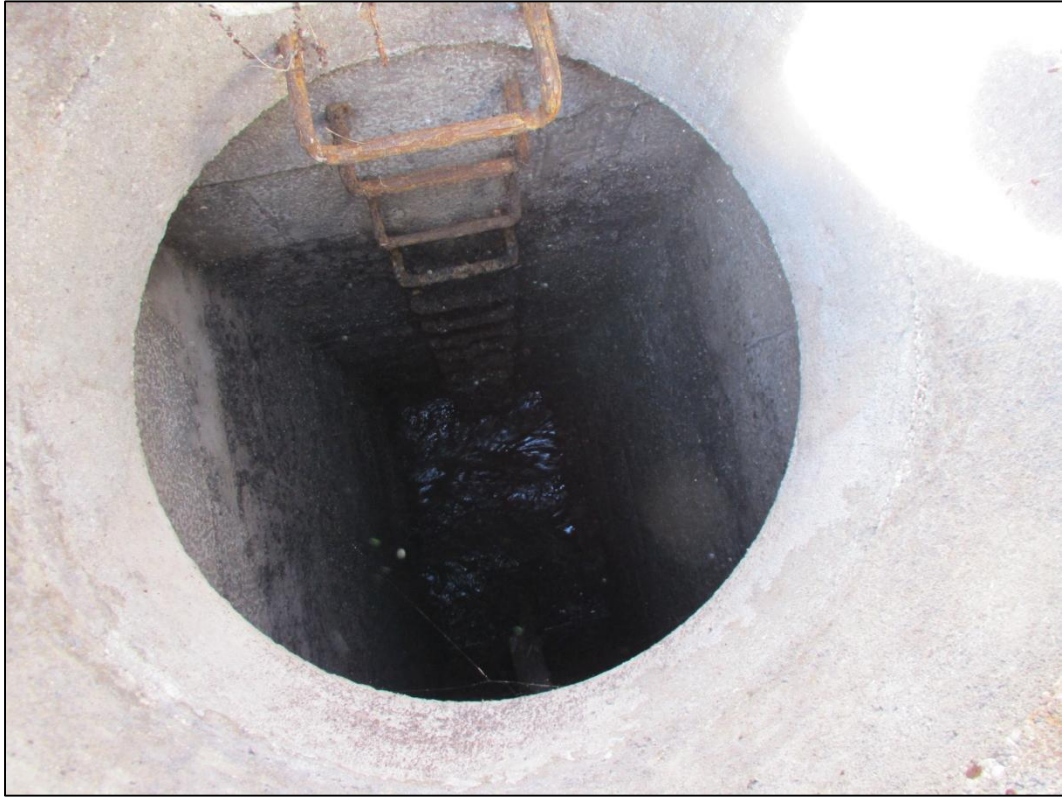
Figure 9 – Chamber access / interior.
