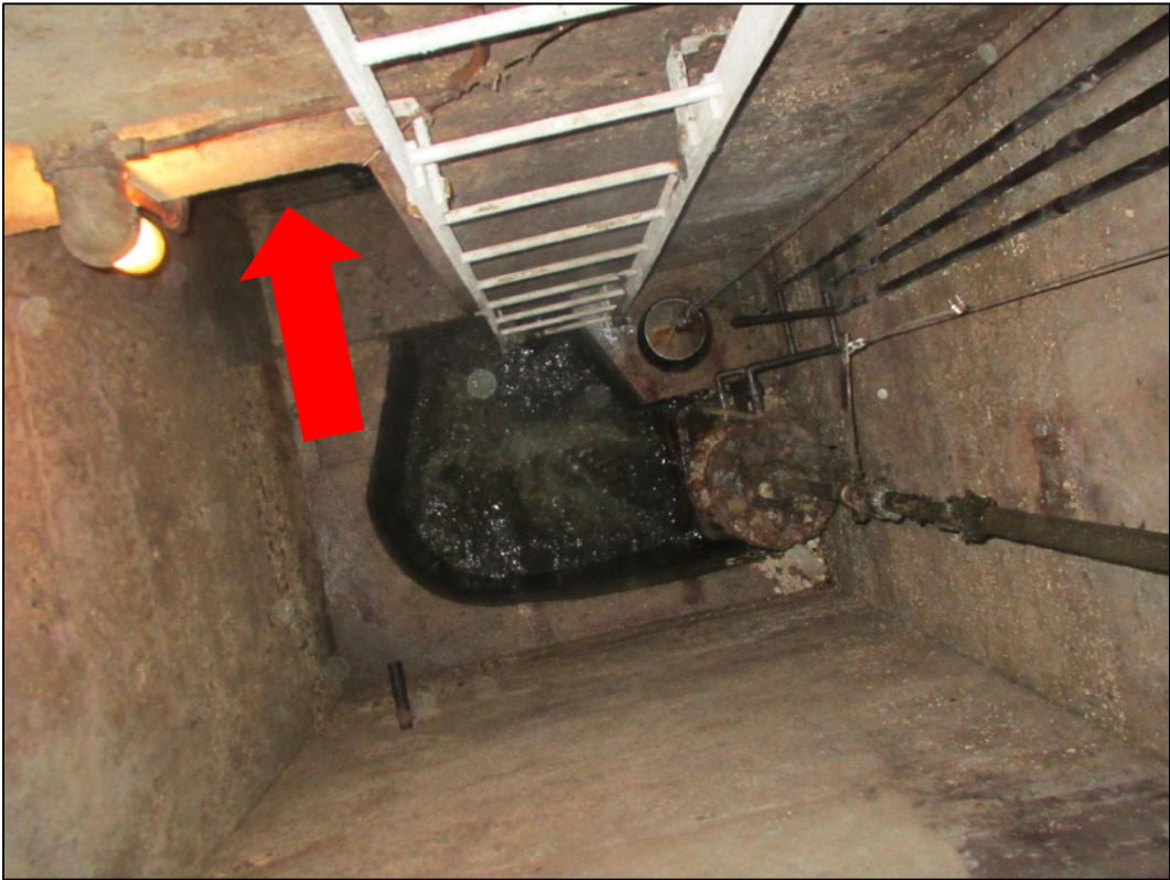
Figure 60 – Bottom sublevel, inlet side of chamber.
