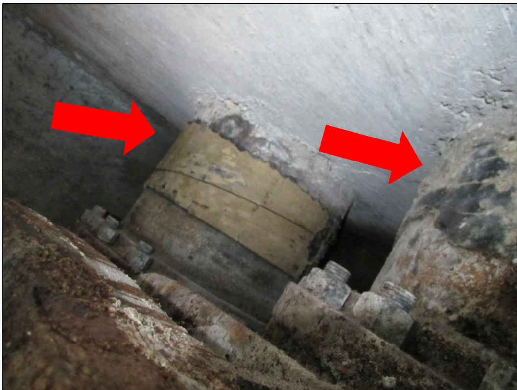
Figure 43 – Pipes exiting downstream wall of chamber.
