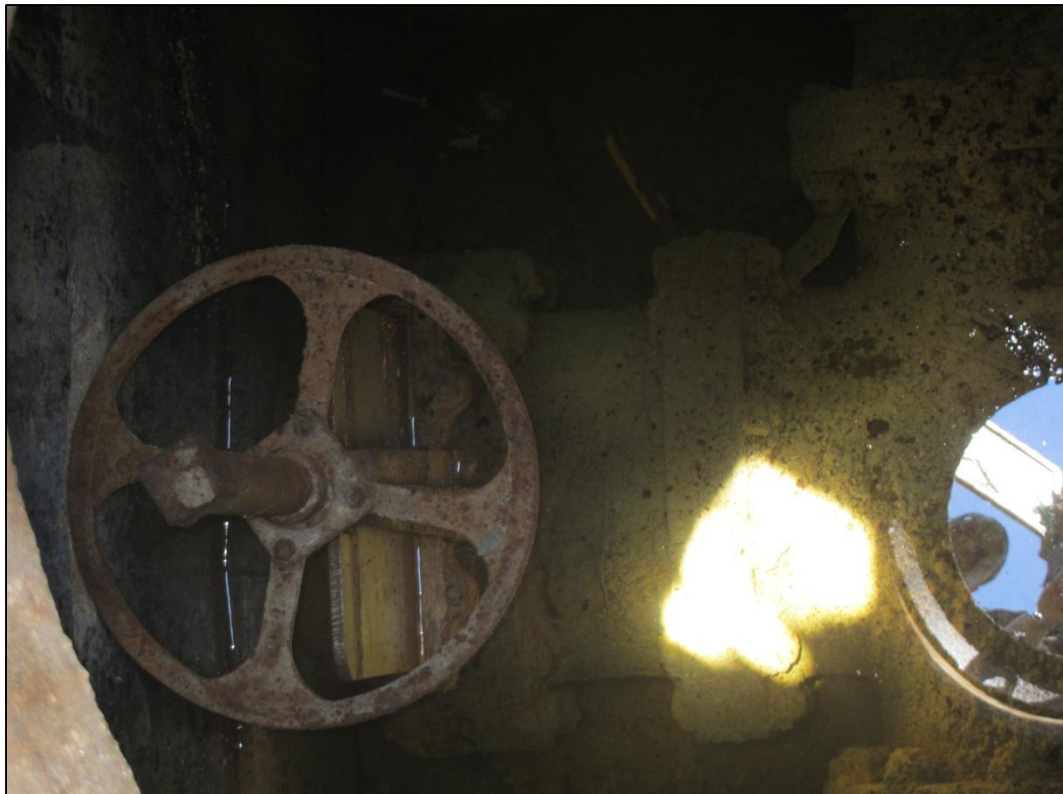
Figure 34 – Knife gate and tee.
