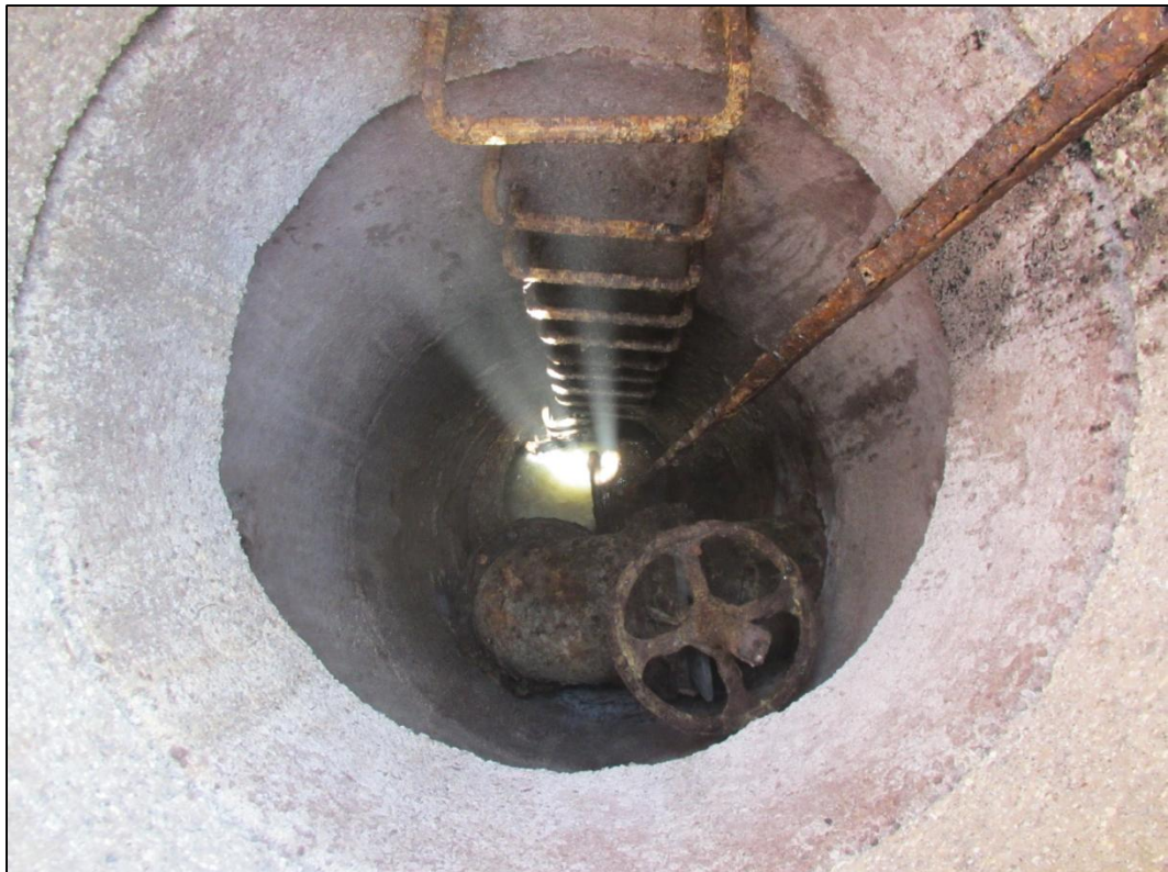
Figure 28 – Chamber access / interior.
