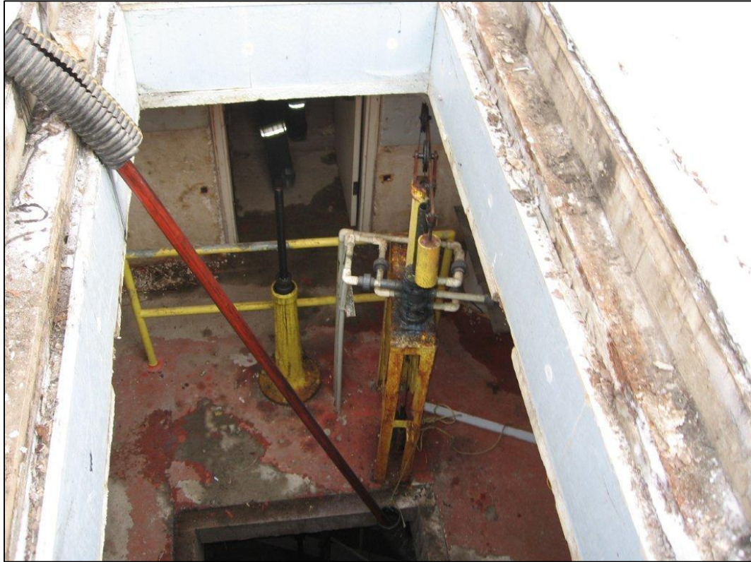
Figure 51 – Main floor opening to first sublevel.
