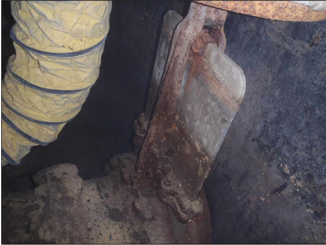
Figure 35 – Knife gate.
