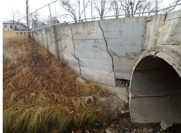
Figure 03 View SE at Wingwall
