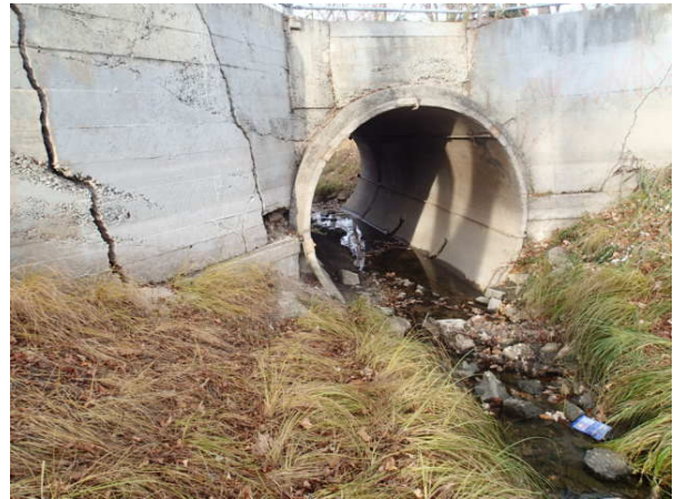
Figure 05 Channel at Outlet of Concrete Pipe
