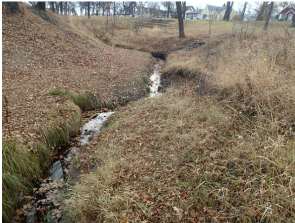
Figure 06 Toe Slump Downstream of Crossing
