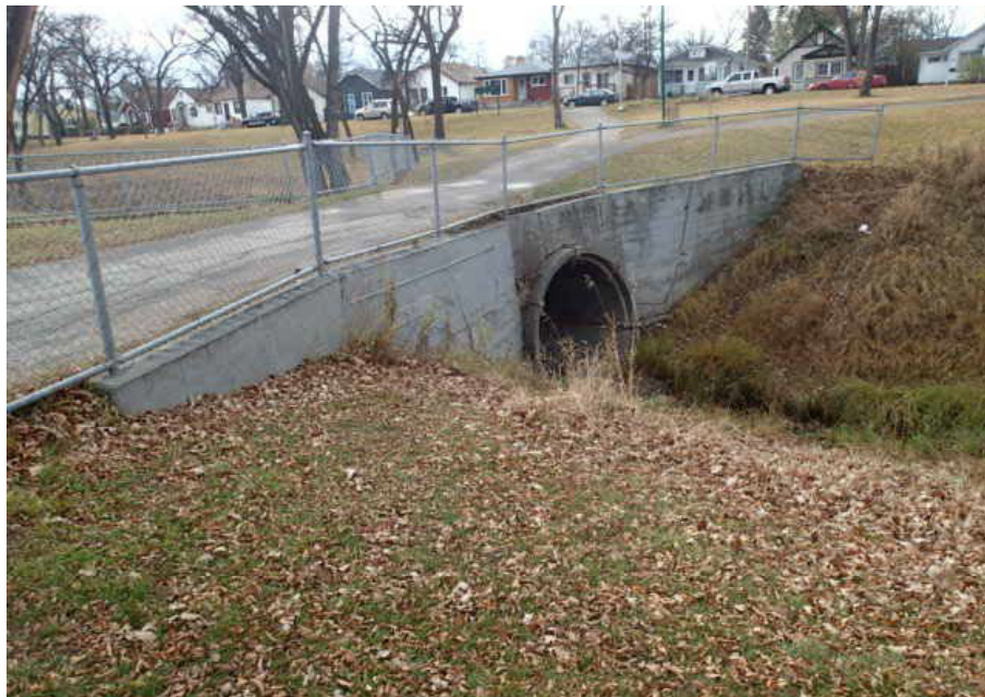
Figure 01 View SE at Crossing
