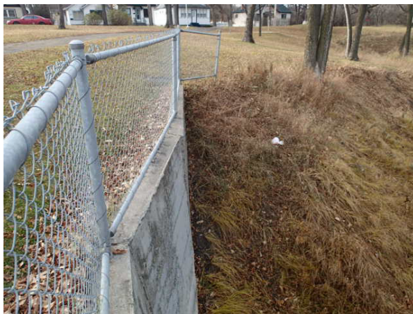
Figure 08 Bank at SW Wingwall
