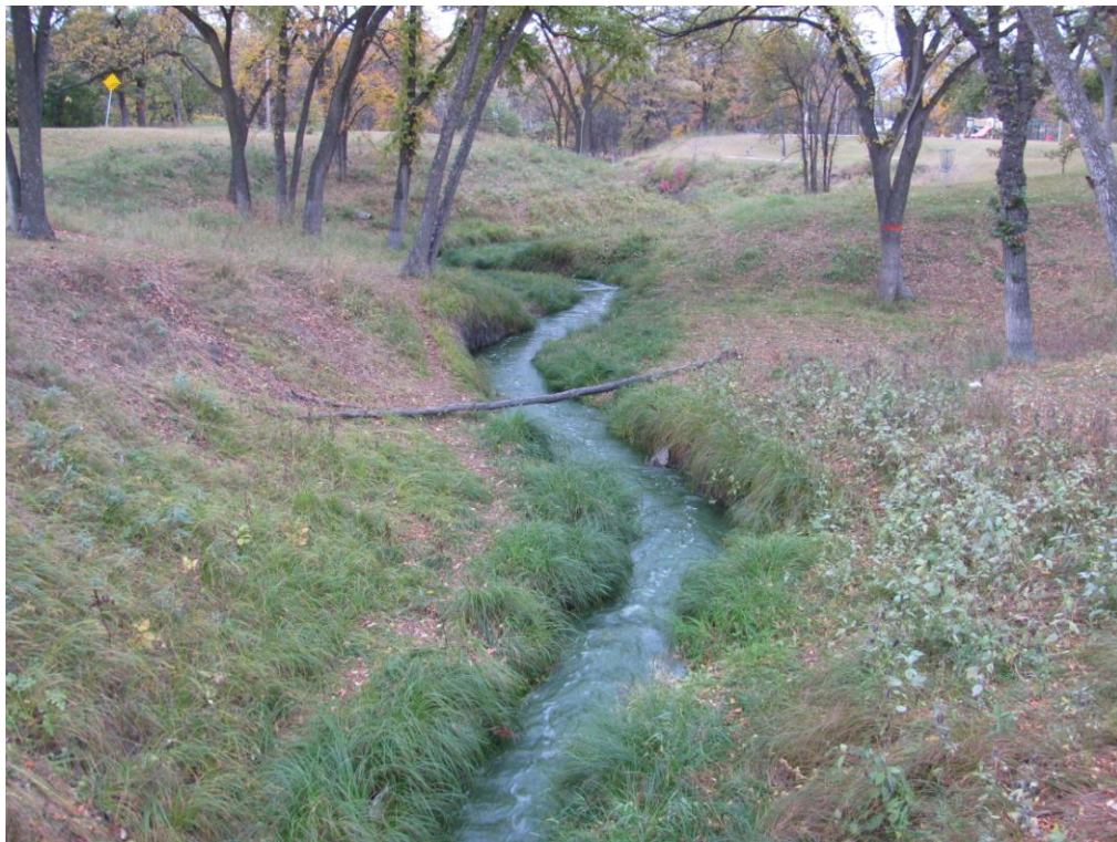
Photo No. 4 Dugald Drain downstream of Happyland Park Crossing
