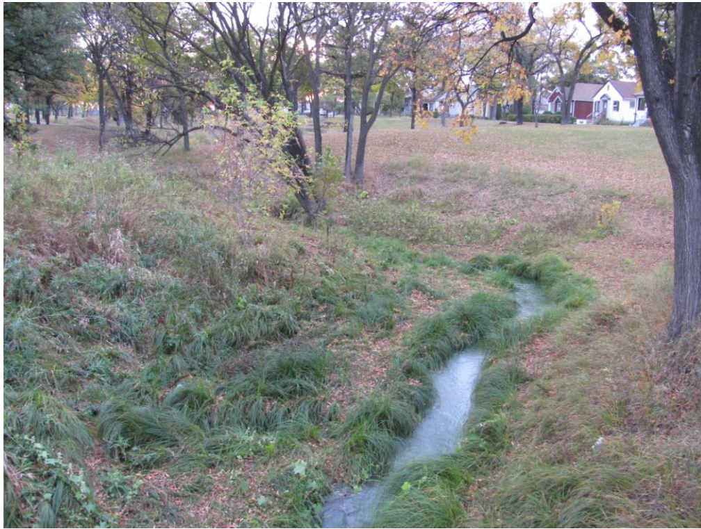
Photo No. 1 Dugald Drain upstream of Happyland Park Crossing
