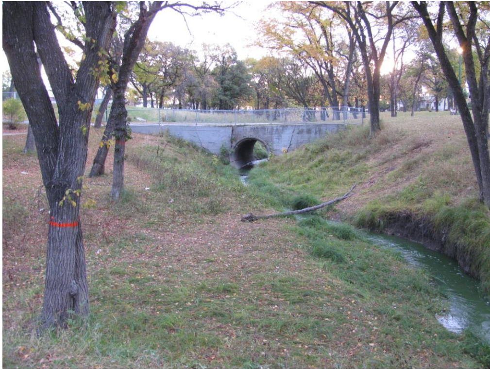
Photo No. 3 Downstream side of Happyland Park Crossing
