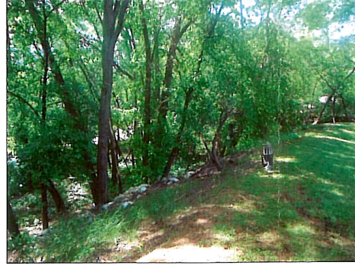
PHOTOGRAPH #5: FACING SOUTH SHOWING TREES NEAR THE EXISTING CLAY DYKE.
