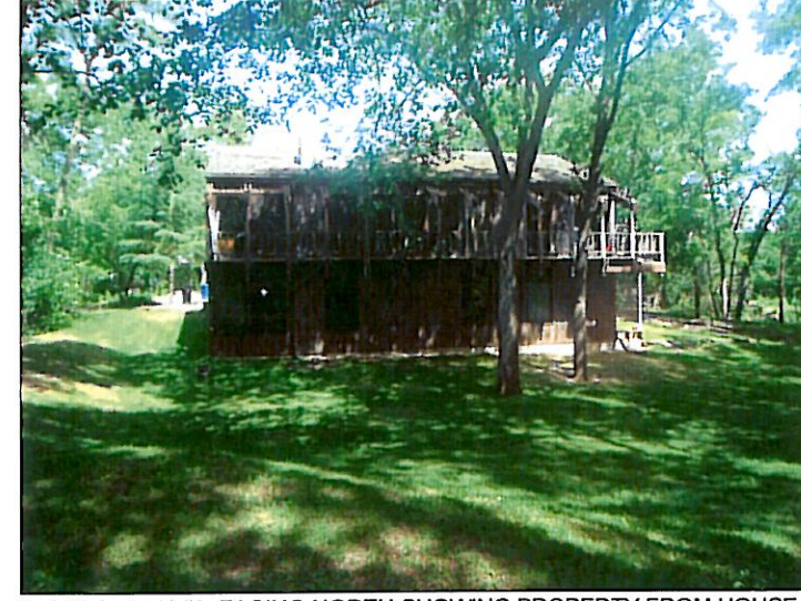
PHOTOGRAPH #3: FACING NORTH SHOWING PROPERTY FROM HOUSE EDGE TO TOP OF CLAY DYKE.
