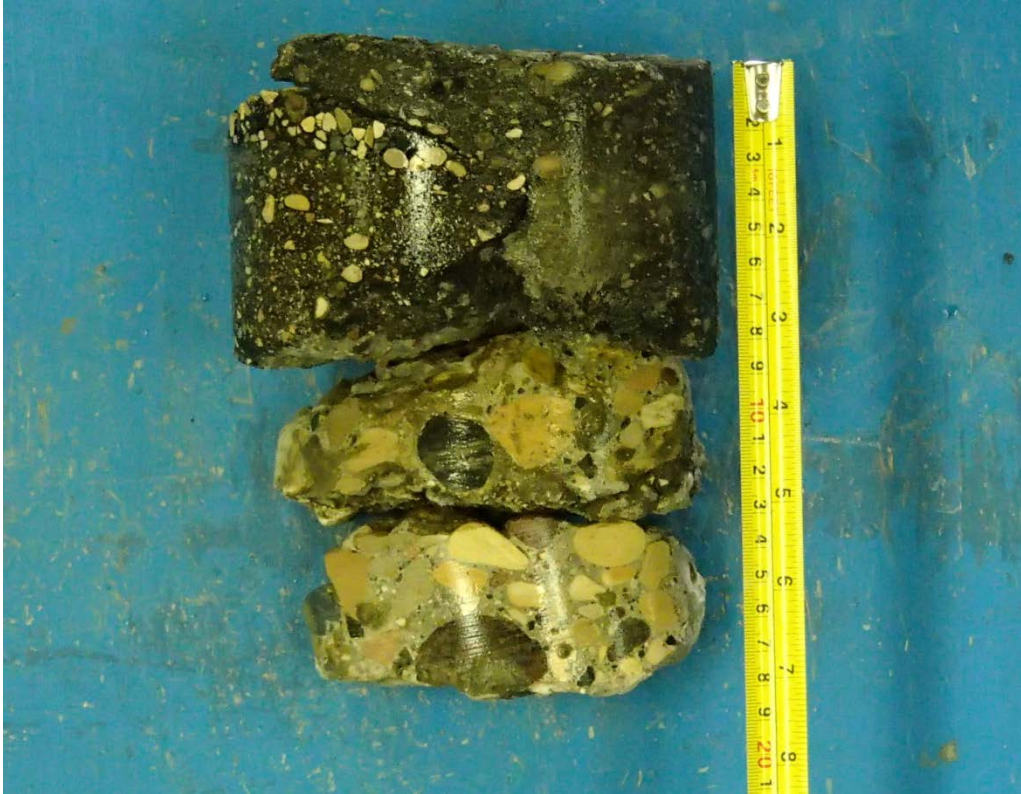
Core sample from Testhole TH1
