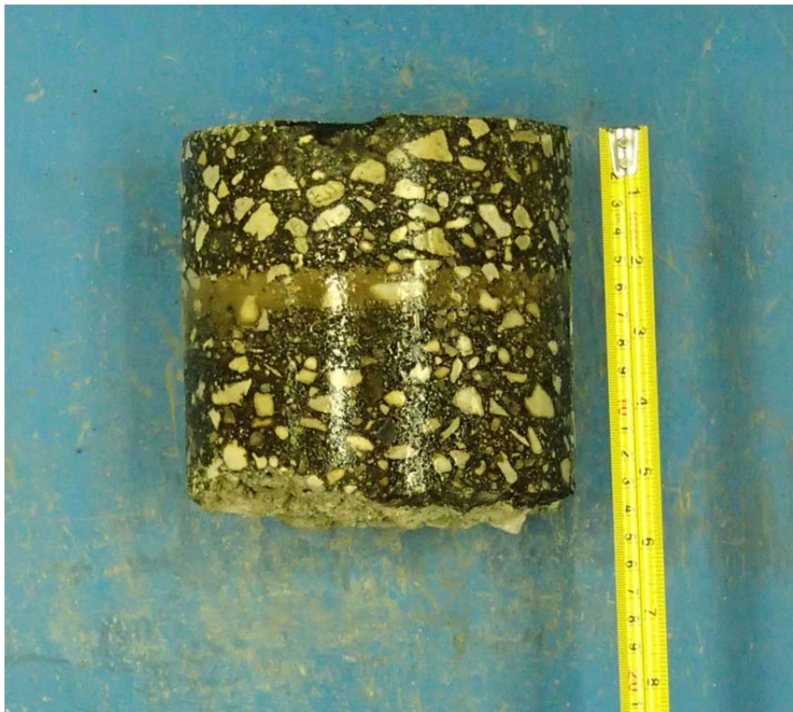
Core sample from Testhole TH2
