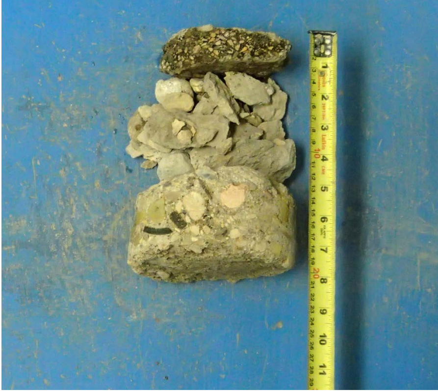
Core sample from Testhole TH1
