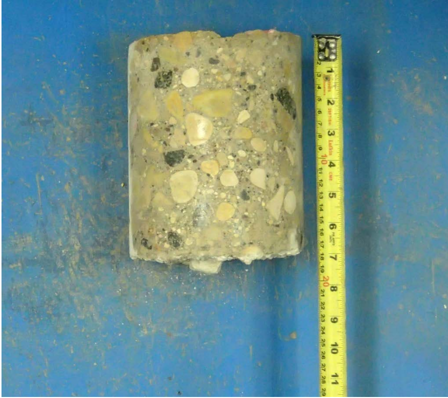
Core sample from Testhole TH3
