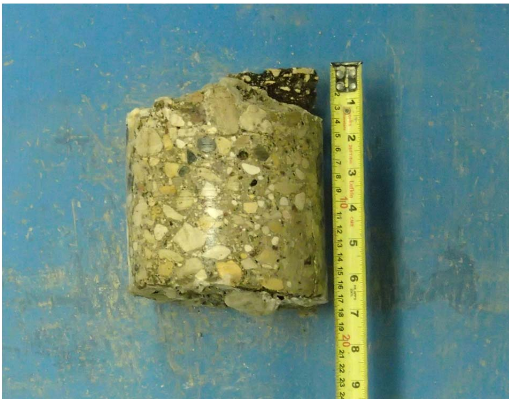
Core sample from Testhole TH8
