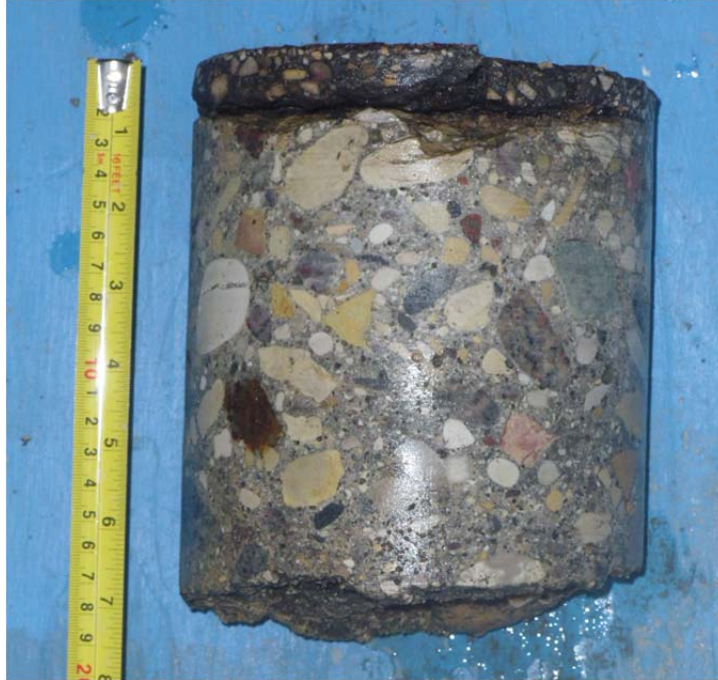
Core sample from Testhole TH5
