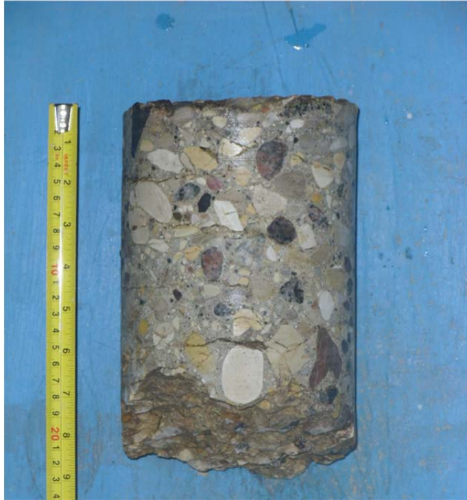
Core sample from Testhole TH5
