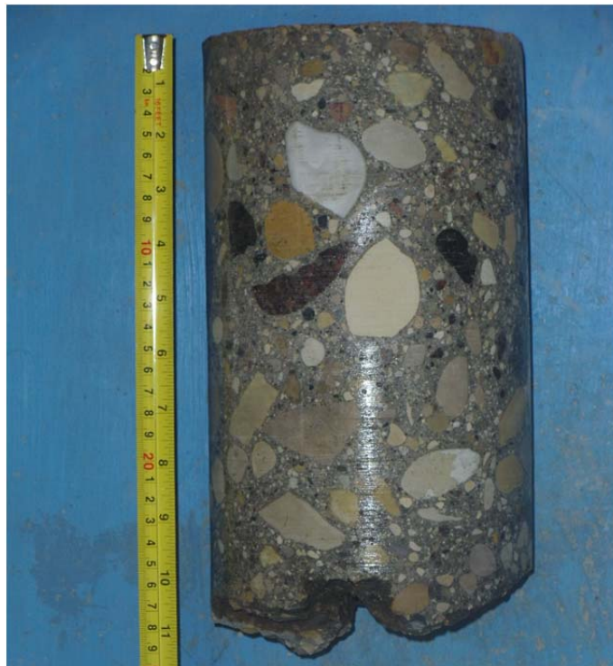
Core sample from Testhole TH2
