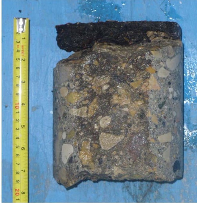
Core sample from Testhole TH3
