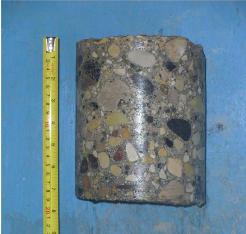
Core sample from Testhole TH1
