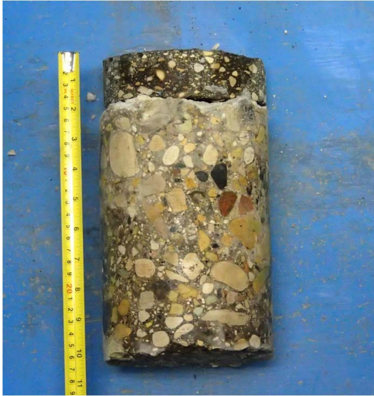
Core sample from Testhole TH5
