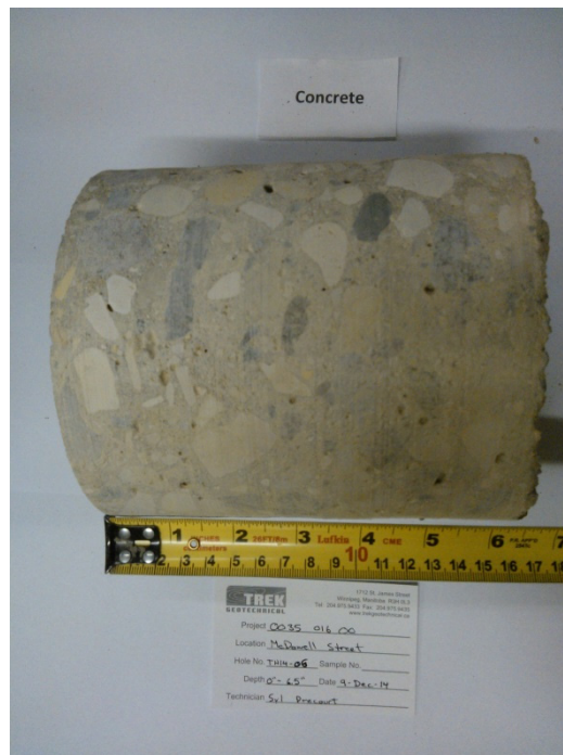
Photo 6: Concrete Core Sample From Test Hole TH14-06
