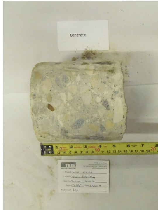
Photo 5: Concrete Core Sample From Test Hole TH14-05
