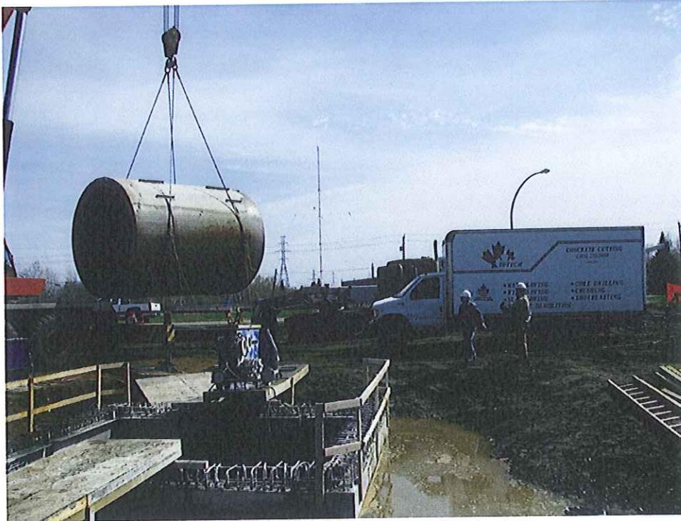
Figure 3 Removal of pipe section at the end of the cut (Thunder Bay, ON)
