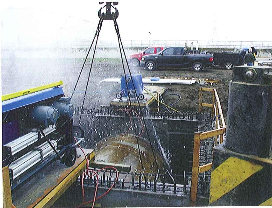
Figure 2 Cutting of large wastewater pipe using a wire saw (Thunder Bay, ON)
