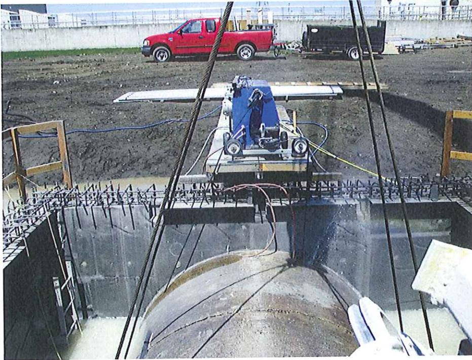
Figure 1 Cutting of a large wastewater pipe using a wire saw under wet conditions (Thunder Bay, ON)
