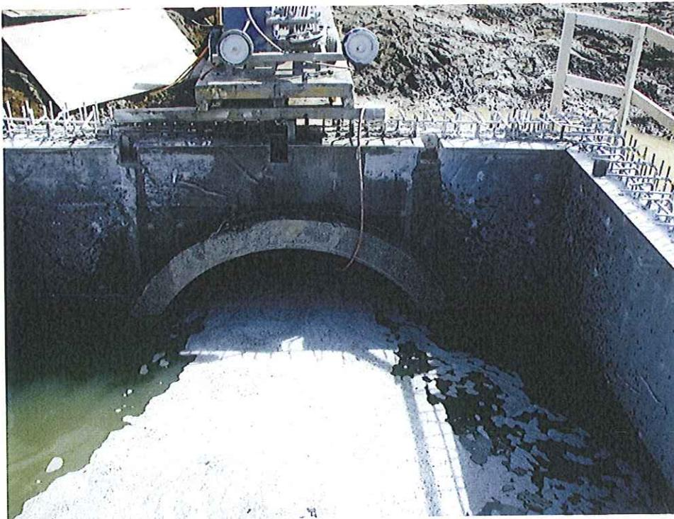
Figure 4 Pipe submerged in wastewater once the cut is completed (Thunder Bay, ON)
