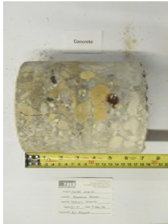
Photo 7: Concrete Core Sample From Test Hole TH14-07
