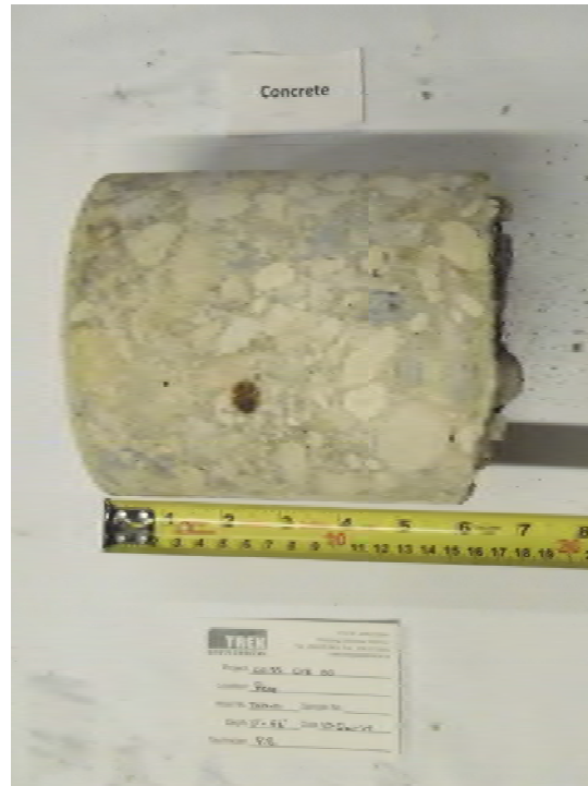
Photo 1: Concrete Core Sample From Test Hole TH14-01
