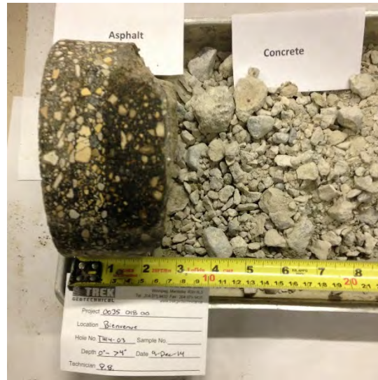
Photo 3: Concrete Core Sample From Test Hole TH14-03
