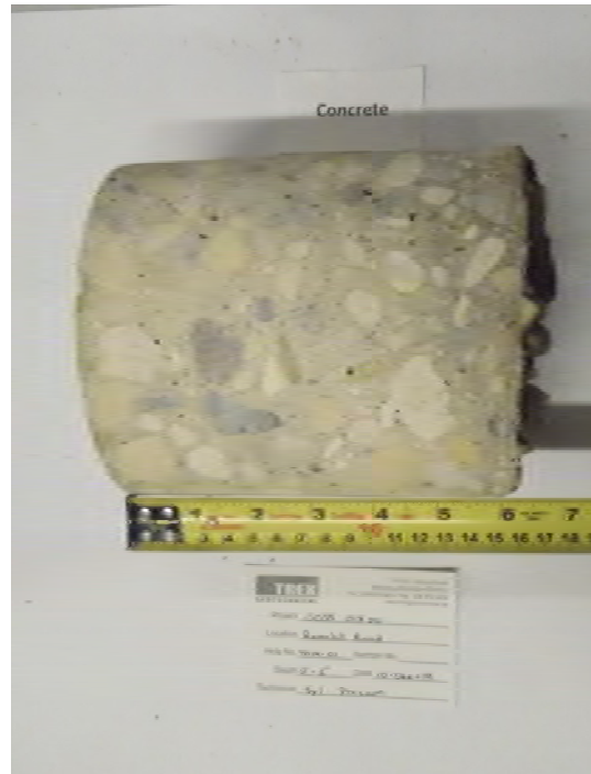
Photo 1: Concrete Core Sample From Test Hole TH14-01
