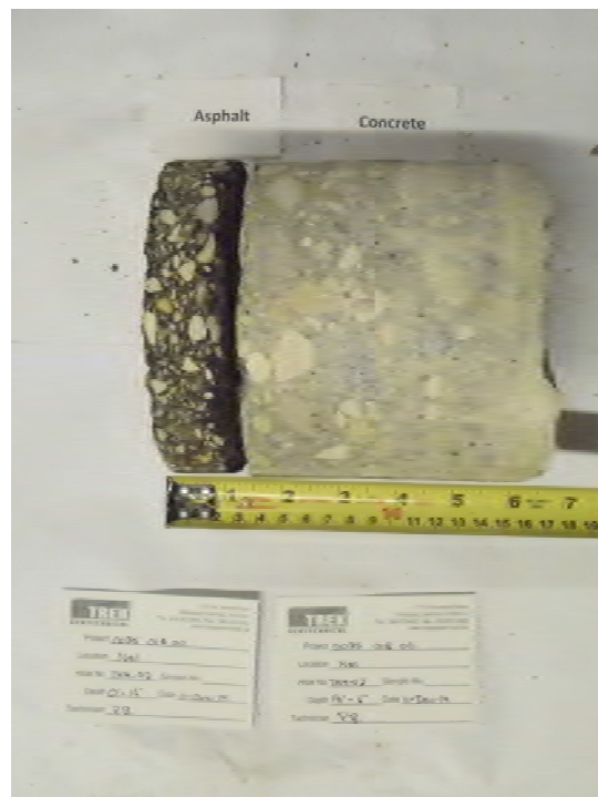
Photo 2: Concrete Core Sample From Test Hole TH14-02
