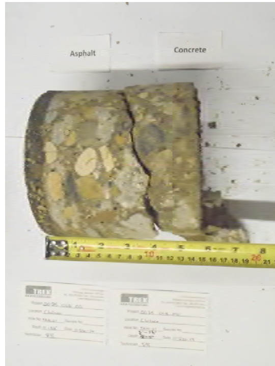
Photo 1: Concrete Core Sample From Test Hole TH14-01
