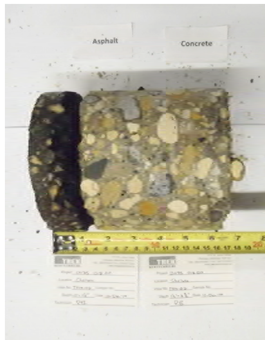
Photo 2: Concrete Core Sample From Test Hole TH14-02
