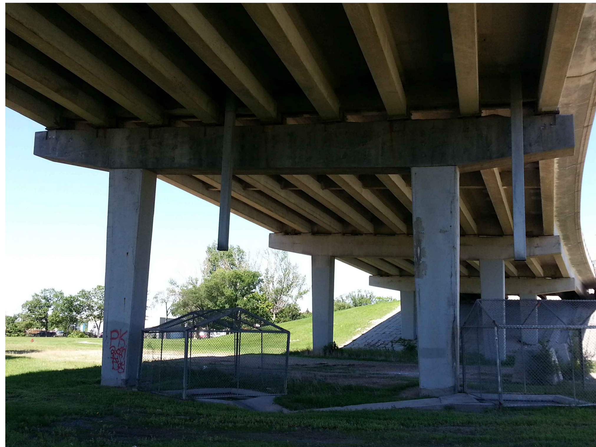
PHOTO - PIER #8 EAST FACE EXISTING CONDITIONS
