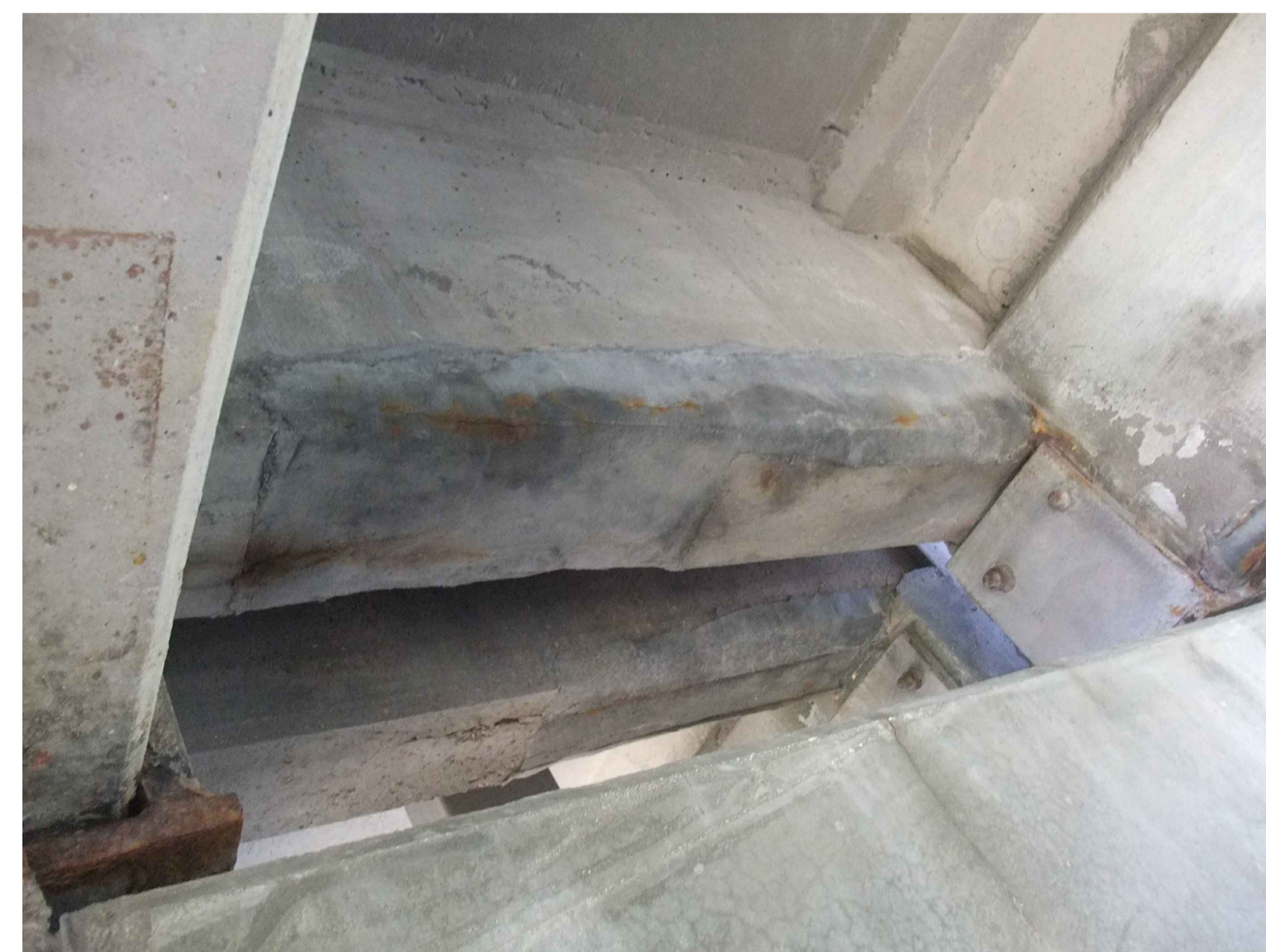
PHOTO - TYPICAL EXISTING CONDITIONS - TYPE 2 REPAIR LOCATION
