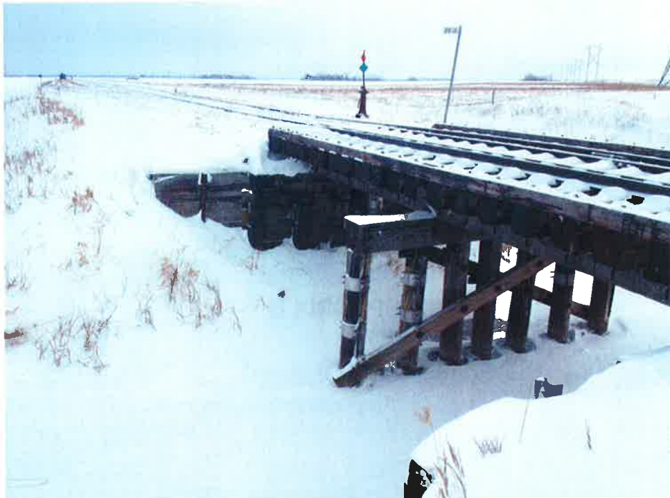
Photo 1: Existing Bridge Foundations, Looking Southeast.
