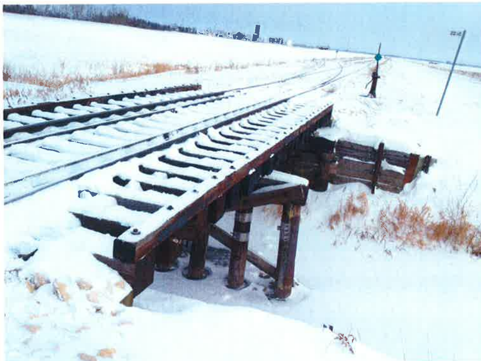
Photo 2: Existing Bridge Foundations, Looking North of east.
