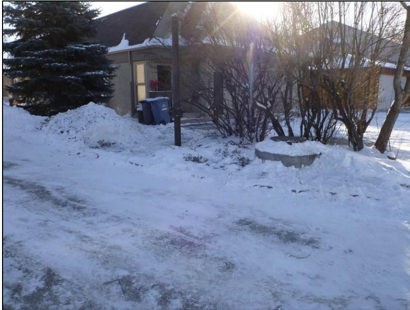
Photograph No. 1 Existing chamber looking southeast
