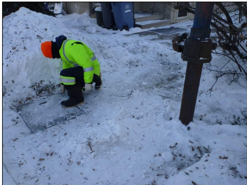
Photograph No. 2 Hatch and gate lift of existing chamber
