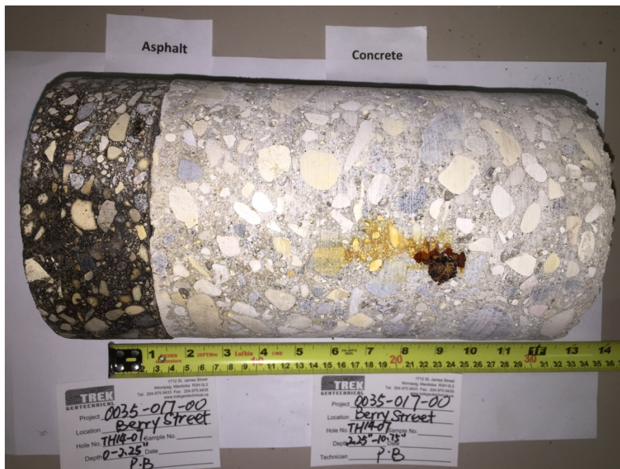
Photo 8: Concrete Core Sample From Test Hole TH14-07
