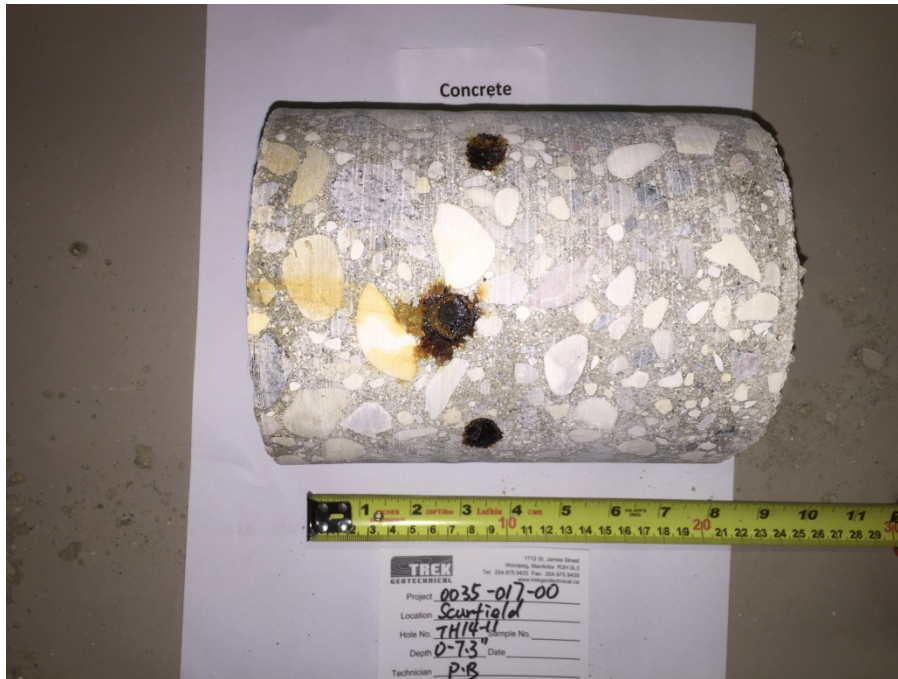
Photo 11: Concrete Core Sample From Test Hole TH14-11
