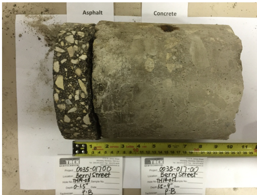
Photo 6: Concrete Core Sample From Test Hole TH14-05
