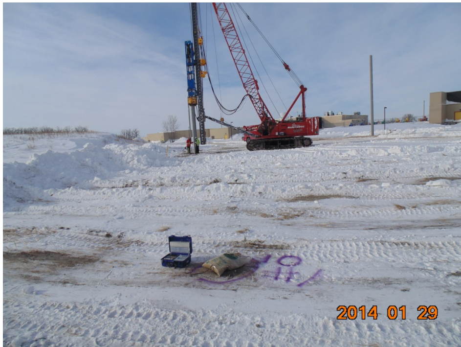
Photo 2 – Pile #1, Showing Monitor M1
