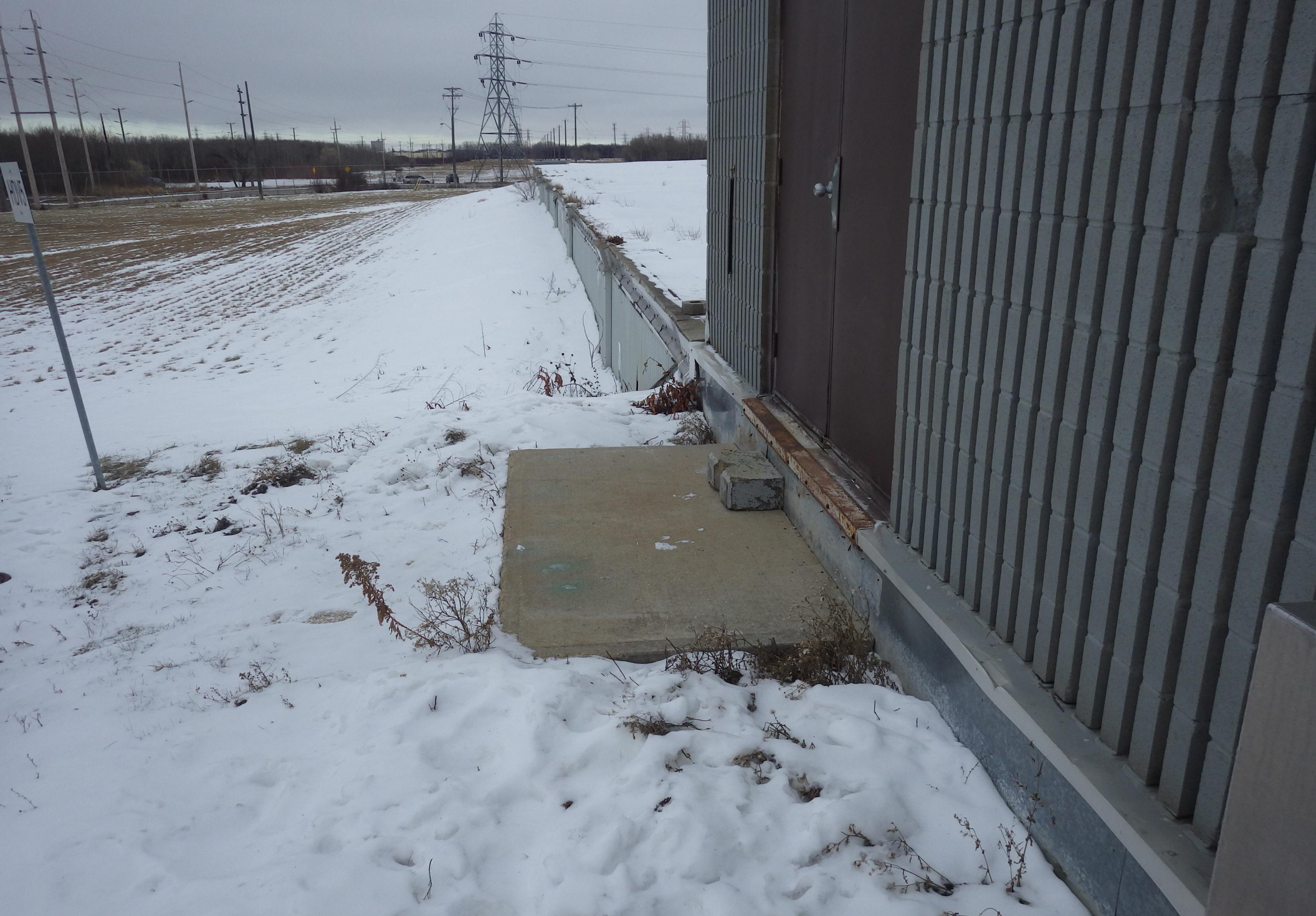
Access Building Slab
