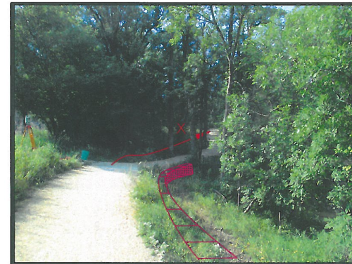
PHOTOGRAPH 6: FACING SOUTH, SHOWING PROPOSED DIVERSION OF WALKWAY. EXISTING TREE AS MARKED TO BE CUT AND DISPOSED. START OF RETAINING WALL ON THE NORTH END IS LOCATED JUST OFF THE PICTURE TO THE RIGHT.
