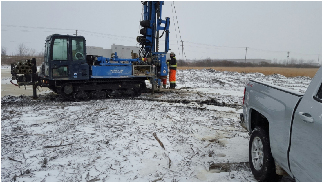
Photo 2: View of drilling operation – November 19, 2015
