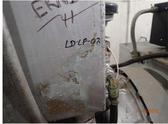
Photo 2. Grey lead-based paint on generator (Sample ID: LD-LP-02).
