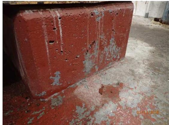
Photo 4. Deep red lead-based paint on floor and generator base (Sample ID: LD-LP-04).
