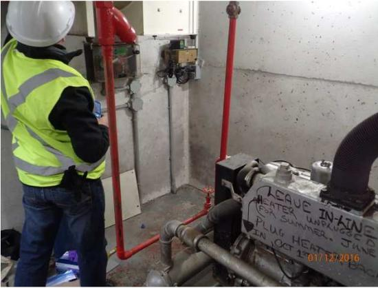
Photo 1. Red lead-based paint on piping (Sample ID: LD-LP-01).
