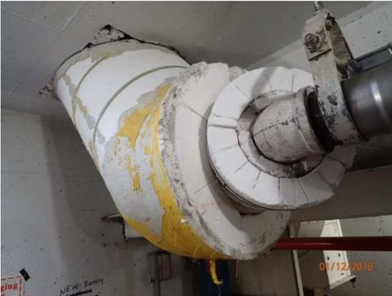
Photo 5. Pipe wrap insulation sampled and analyzed for asbestos content.
