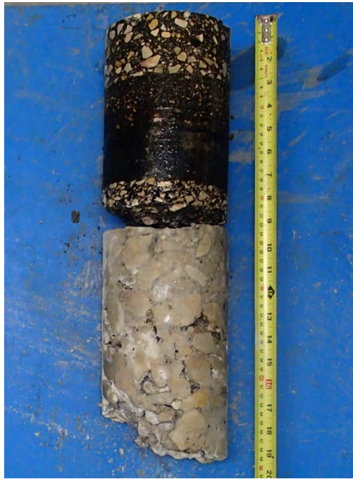
Photo 11 – Core sample from Testhole TH11
