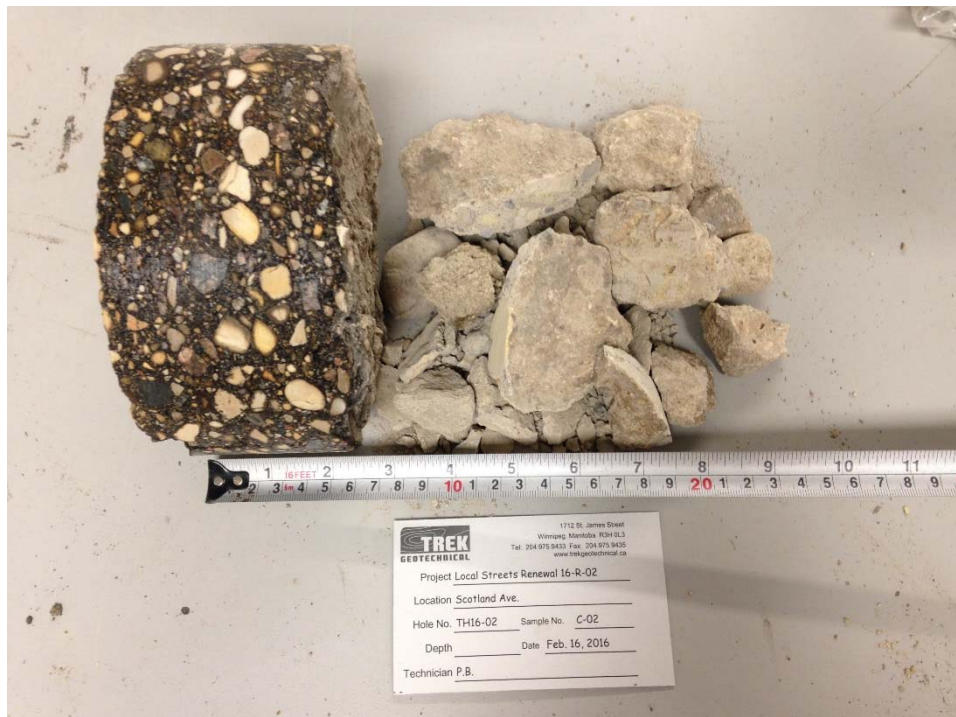
Photo 2: Pavement Core Sample at Test Hole TH16-02
