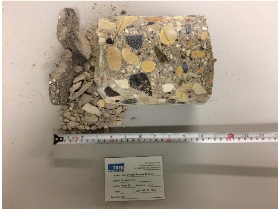
Photo 1: Pavement Core Sample at Test Hole TH16-01
