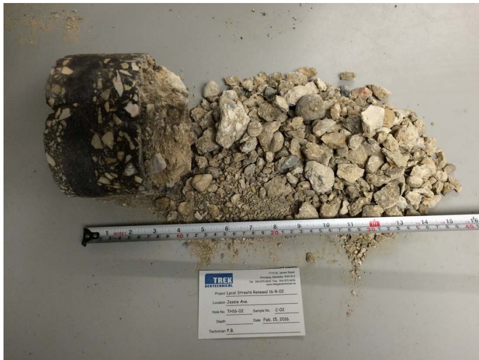
Photo 2: Pavement Core Sample at Test Hole TH16-02
