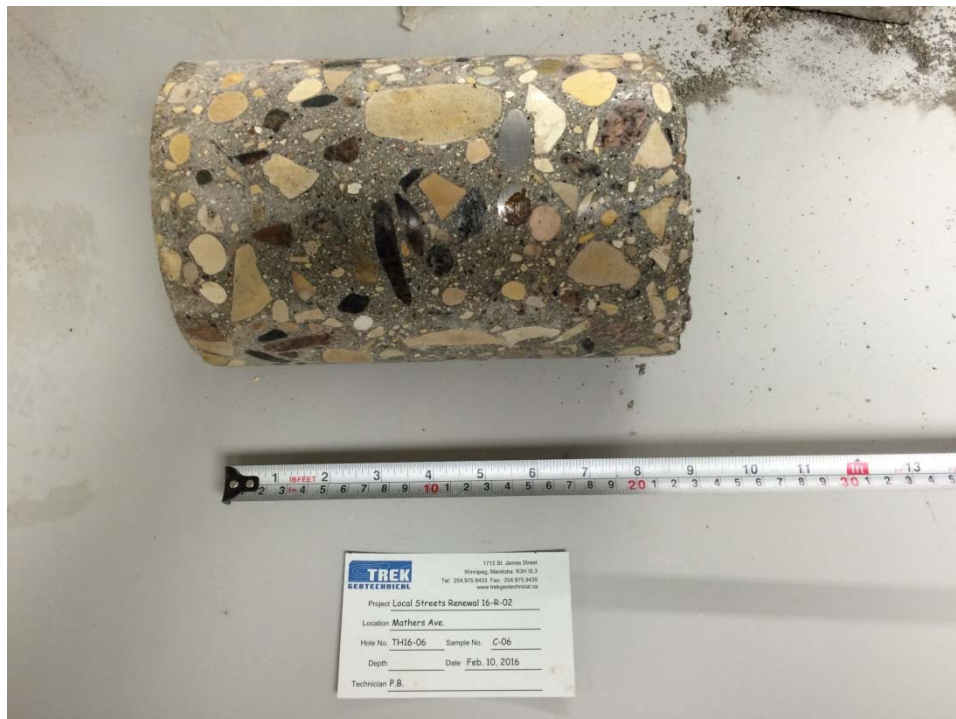
Photo 6: Pavement Core Sample at Test Hole TH16-06
