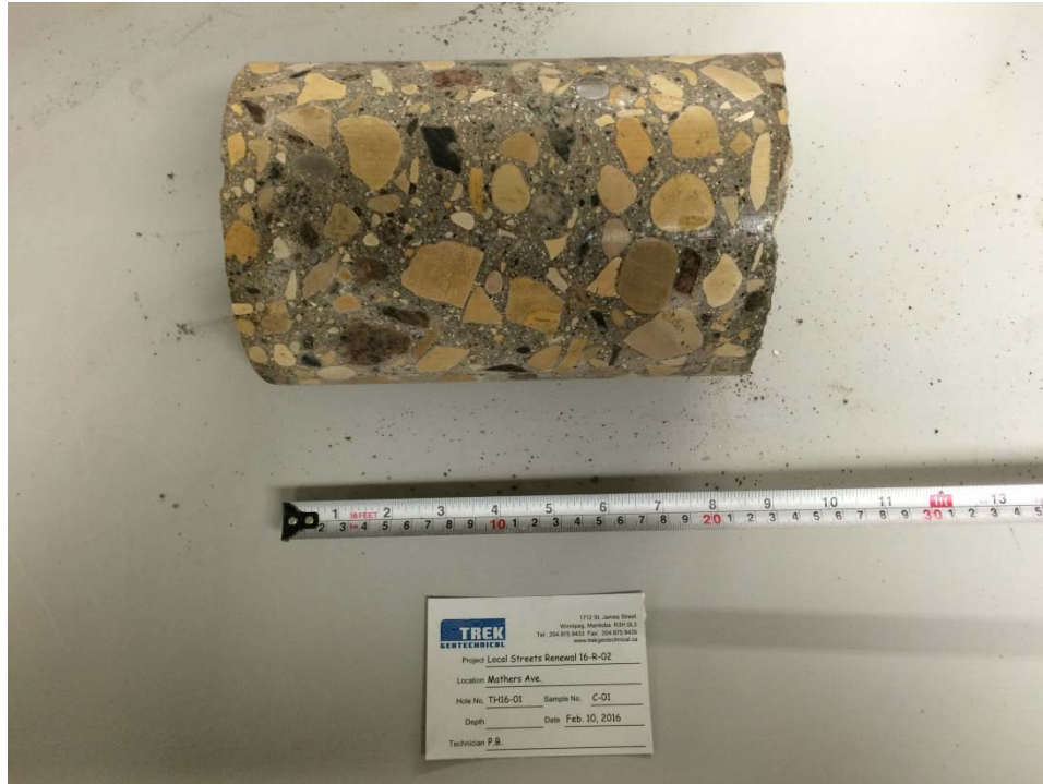
Photo 1: Pavement Core Sample at Test Hole TH16-01
