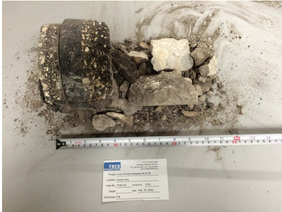
Photo 1: Pavement Core Sample at Test Hole TH16-01
