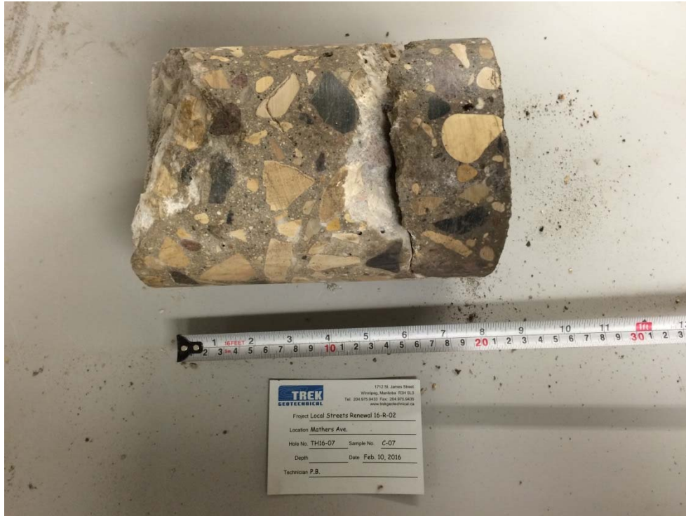
Photo 7: Pavement Core Sample at Test Hole TH16-07
