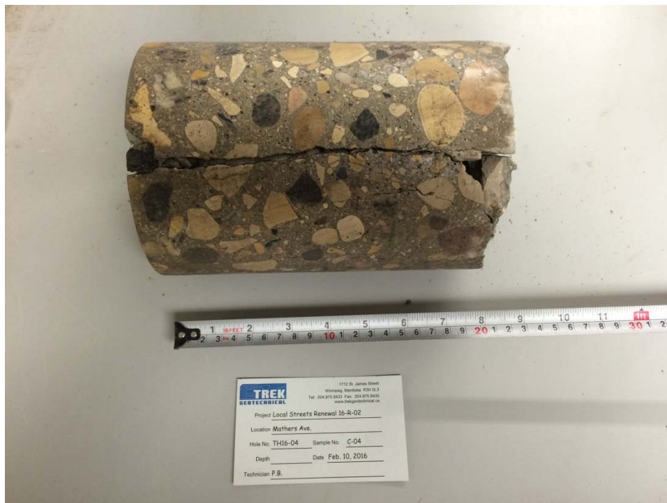
Photo 4: Pavement Core Sample at Test Hole TH16-04
