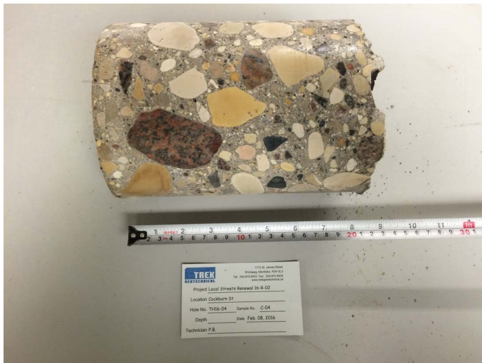
Photo 4: Pavement Core Sample at Test Hole TH16-04
