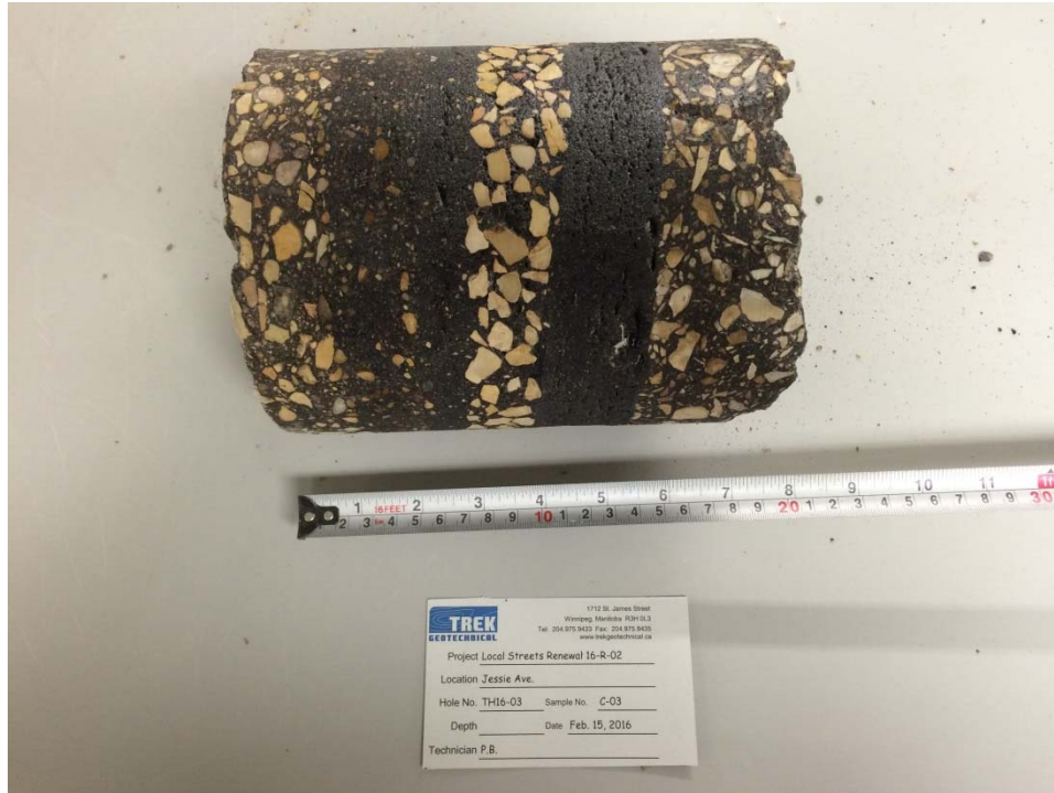
Photo 3: Pavement Core Sample at Test Hole TH16-03
