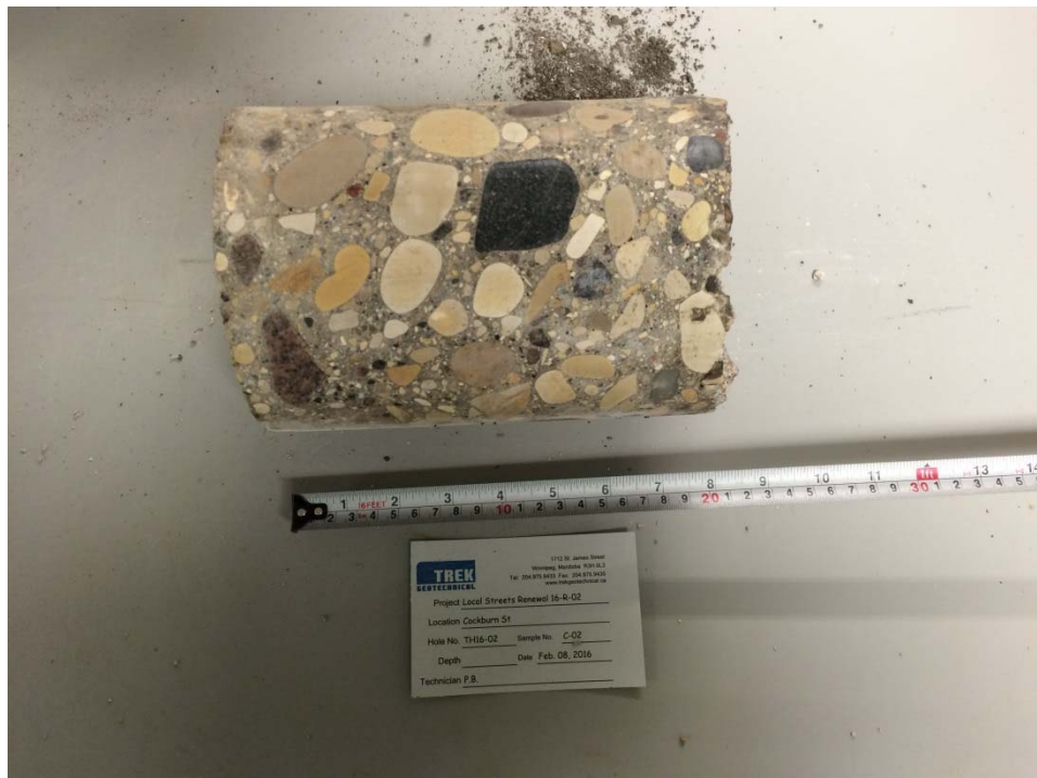
Photo 2: Pavement Core Sample at Test Hole TH16-02
