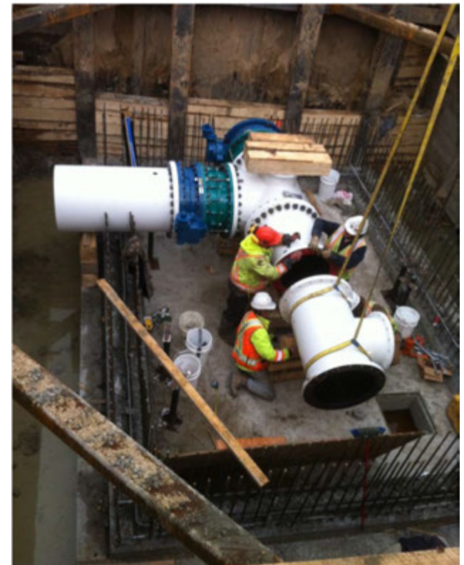
Eldridge & Haney valve chamber replacements
