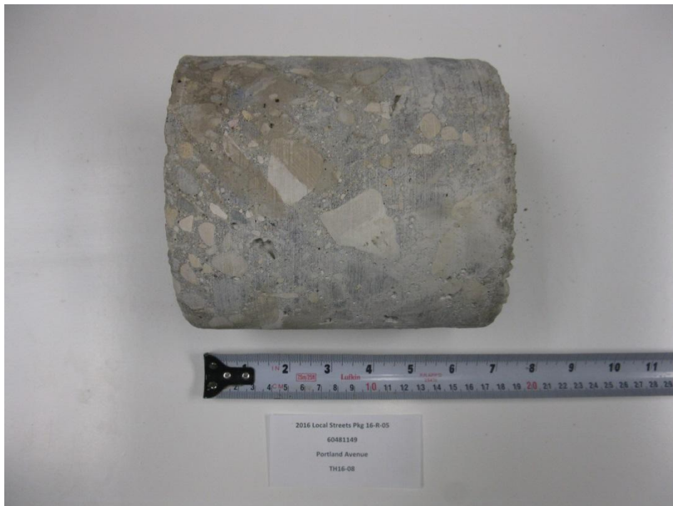
Photograph 8. Portland Avenue – TH16-08
