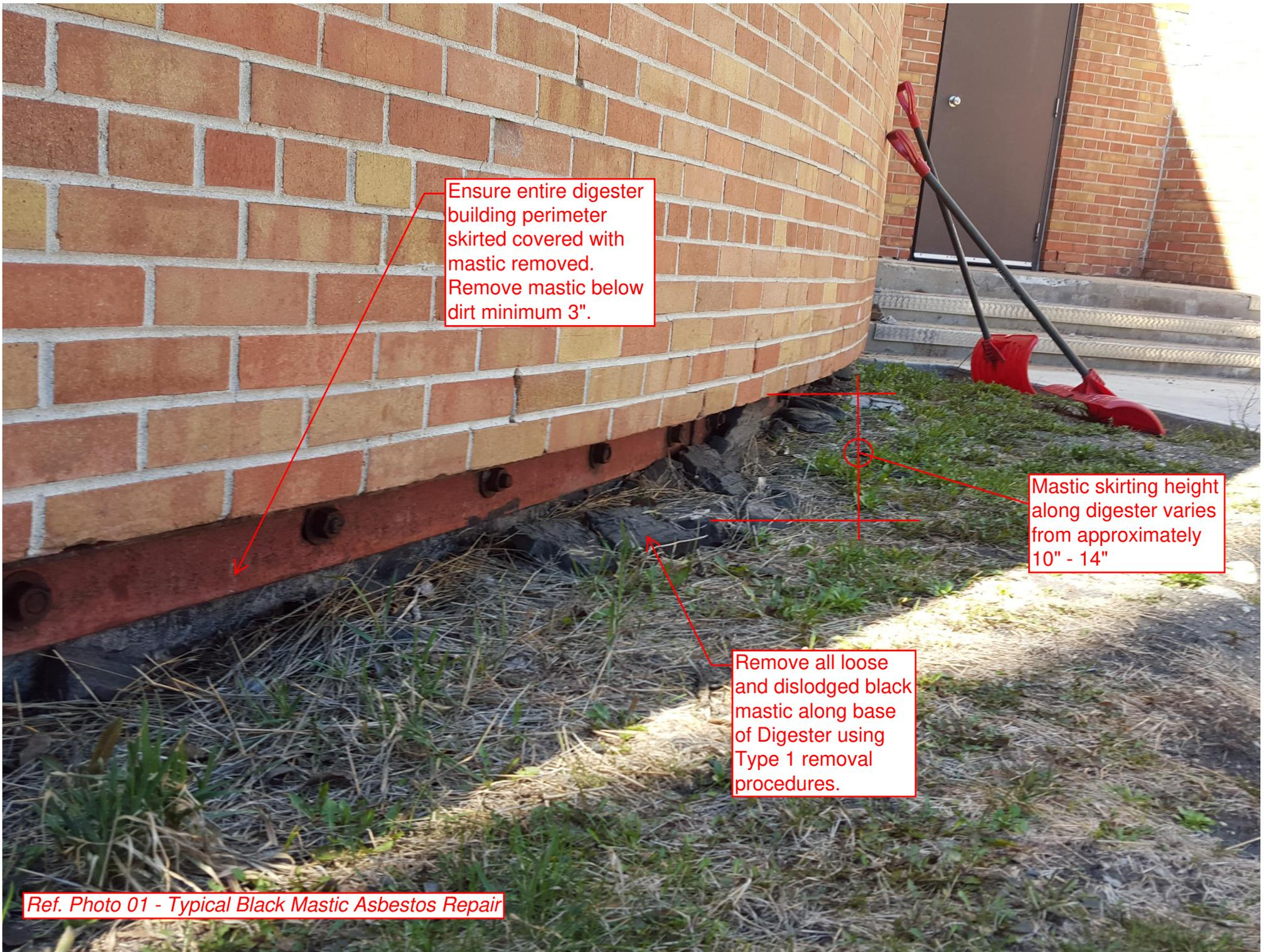
Ensure entire digester building perimeter skirted covered with mastic removed. Remove mastic below dirt minimum 3".
