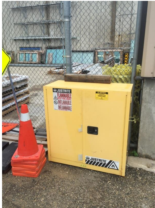
Photo 5. Flammable liquid storage cabinet lock box adjacent to Storage Shed.
