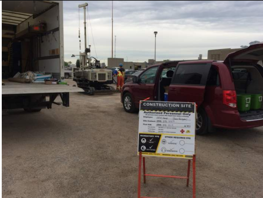
Photo 5. Work area for BH04, construction site sign in place to raise public awareness to safety concerns.
