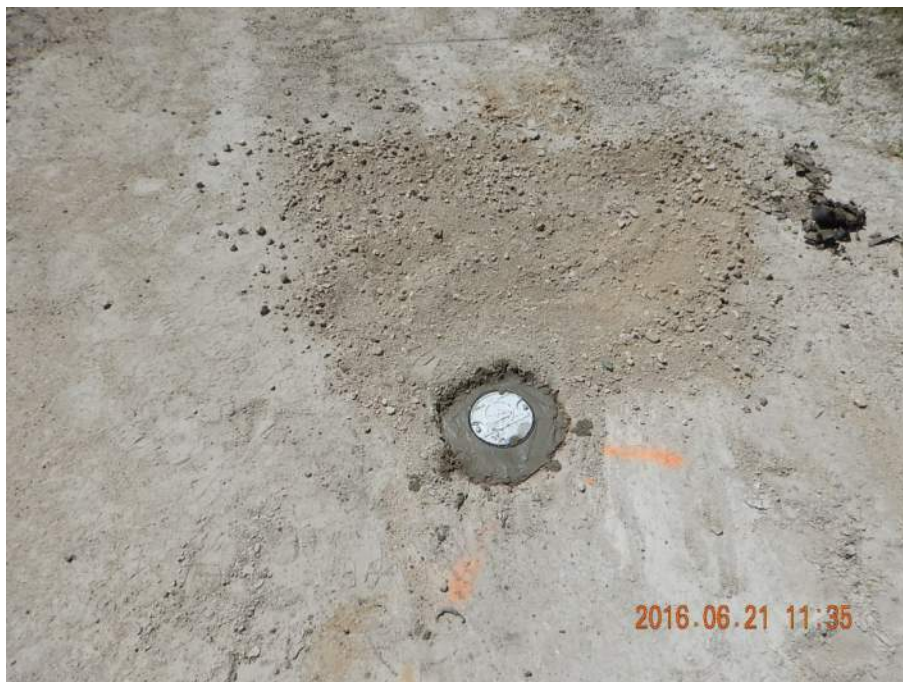
Photo 4. Flush mount well cover, cemented in place in the parking lot at 421 Osborne Street.
