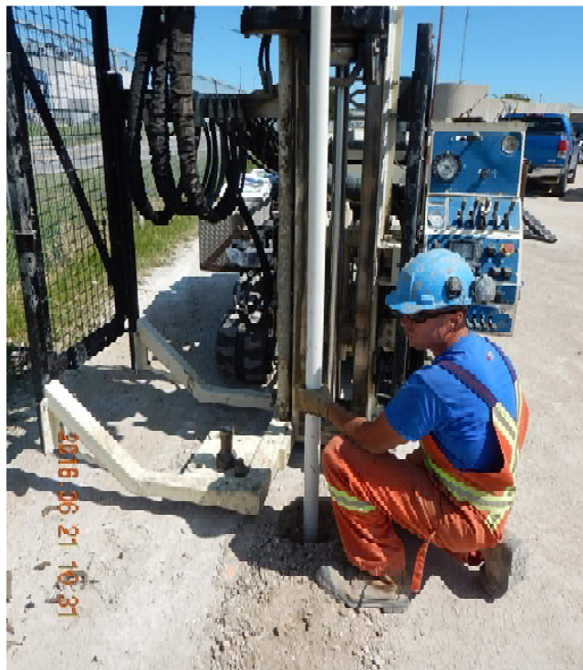
Photo 2. Monitoring well (MW05) installation by Maple Leaf.
