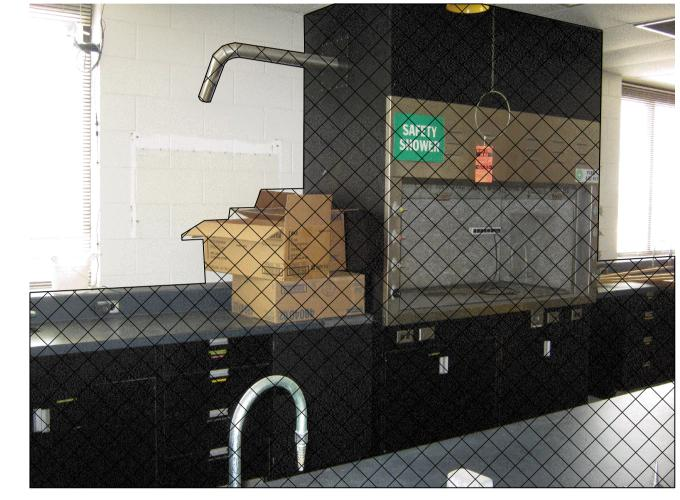
EXISTING WORKSTATION/ MILLWORK TO BE REMOVED. EXISTING FUME HOOD TO BE REMOVED & DISCONNECTED. NOTE 6.
