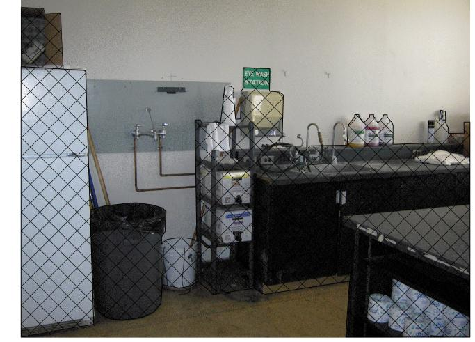
EXISTING EQUIPMENTS & WORKSTATION/ MILLWORK TO BE REMOVED. EXISTING WALL-MOUNTED FAUCET TO REMAIN. EXISTING SINK TO BE REMOVED. REFER TO MECHANICAL DRAWINGS.
