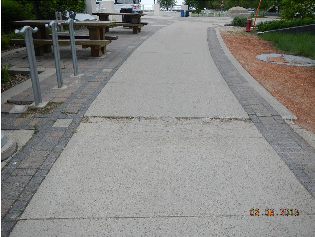
West Abutment Plaza - Location 2
