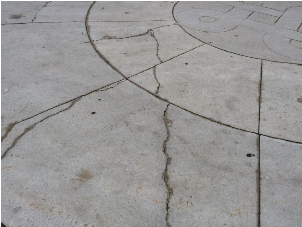
West Abutment Plaza - Location 3
