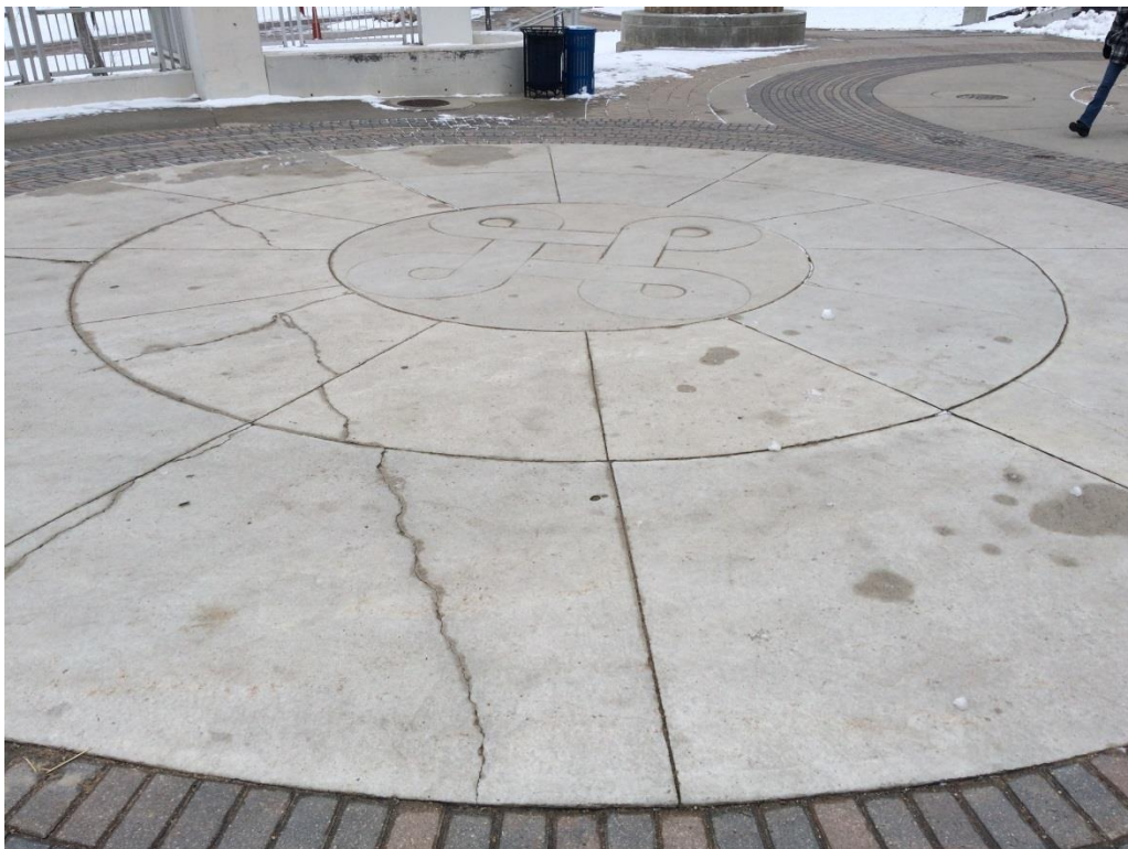
West Abutment Plaza - Location 3
