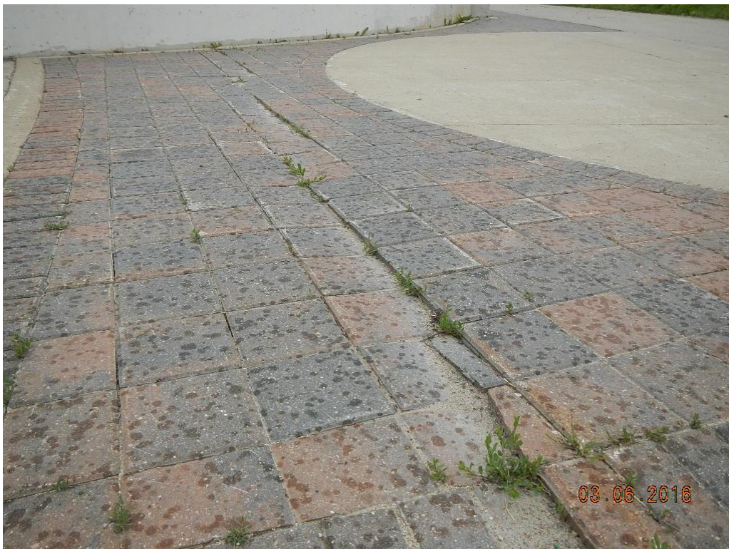
West Abutment Plaza - Location 3
