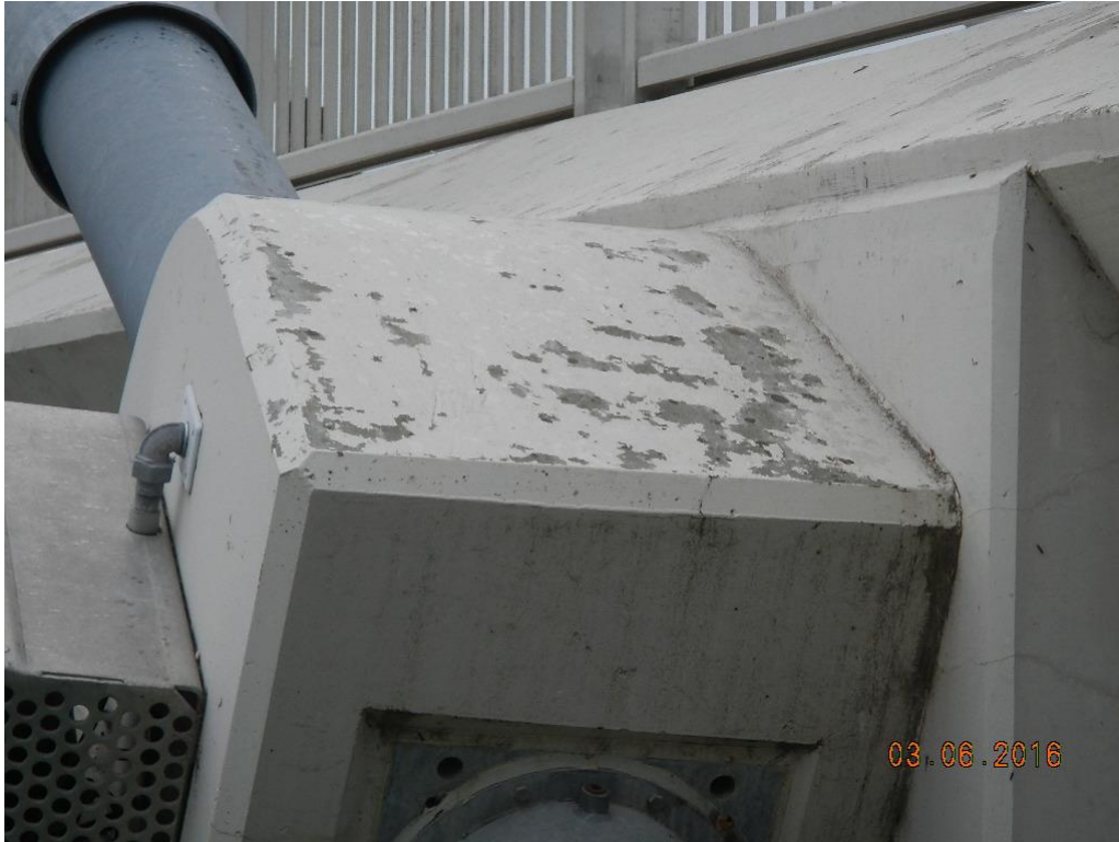
Painting Limits - Concrete Anchor Blocks
