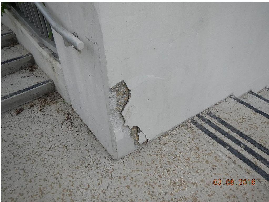
West Abutment Plaza - Location 1
