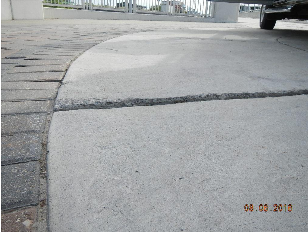
West Abutment Plaza - Location 3
