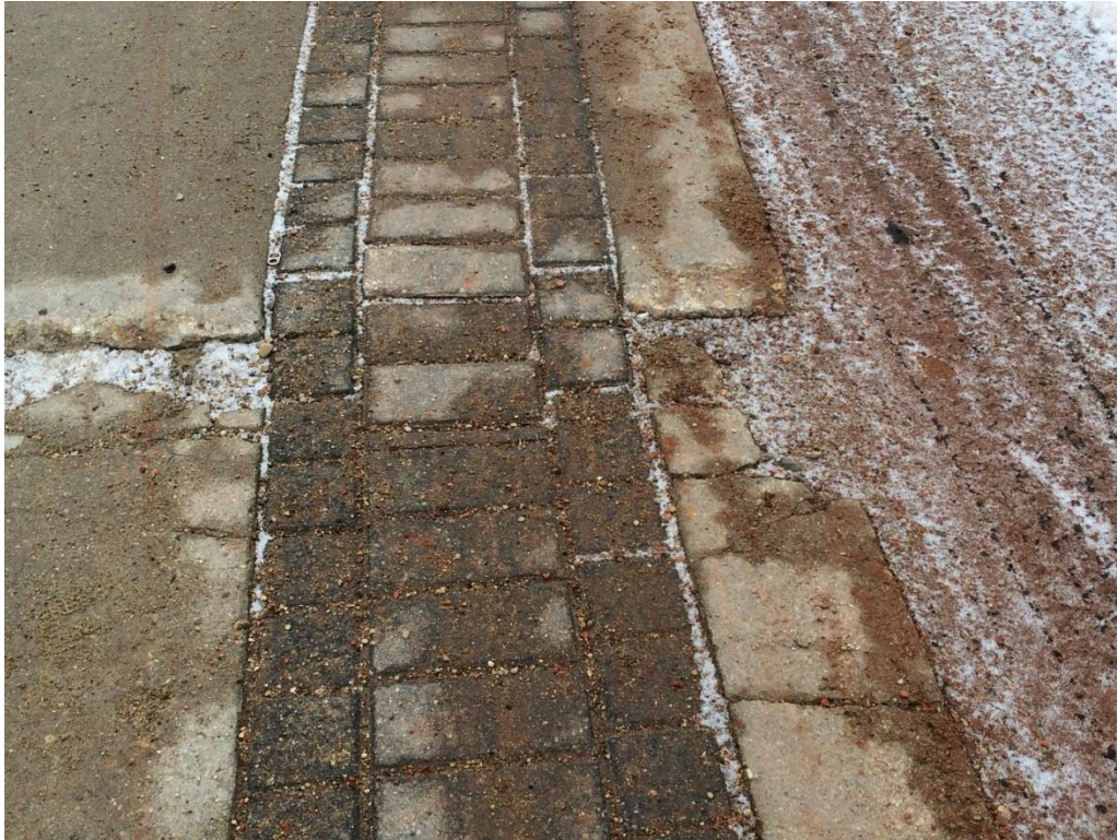
West Abutment Plaza - Location 2
