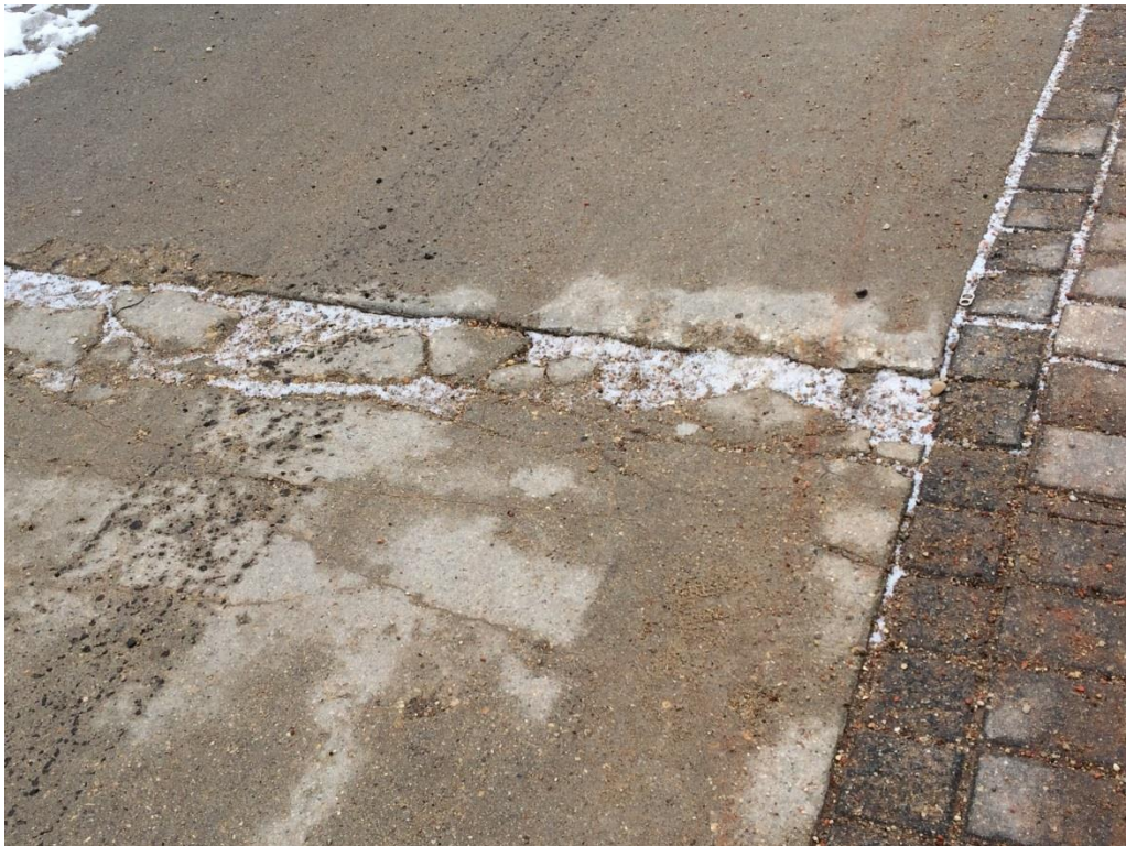
West Abutment Plaza - Location 2
