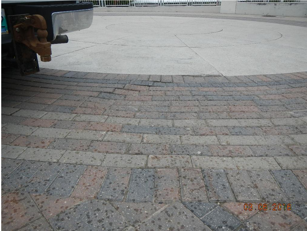
West Abutment Plaza - Location 3
