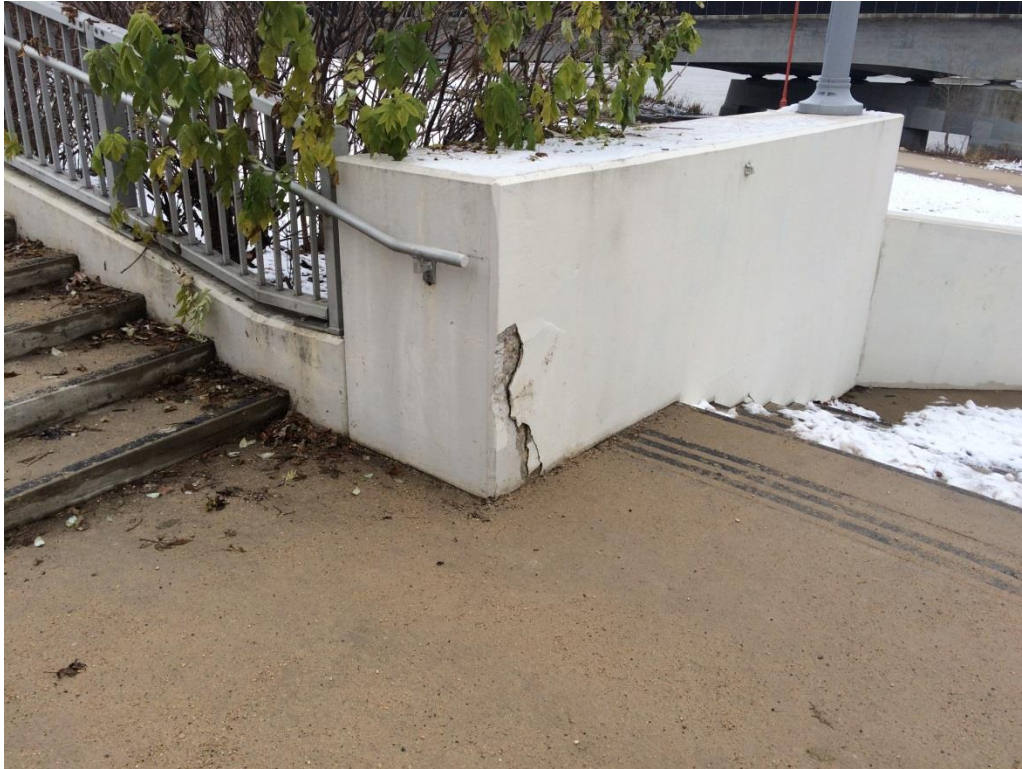
West Abutment Plaza - Location 1
