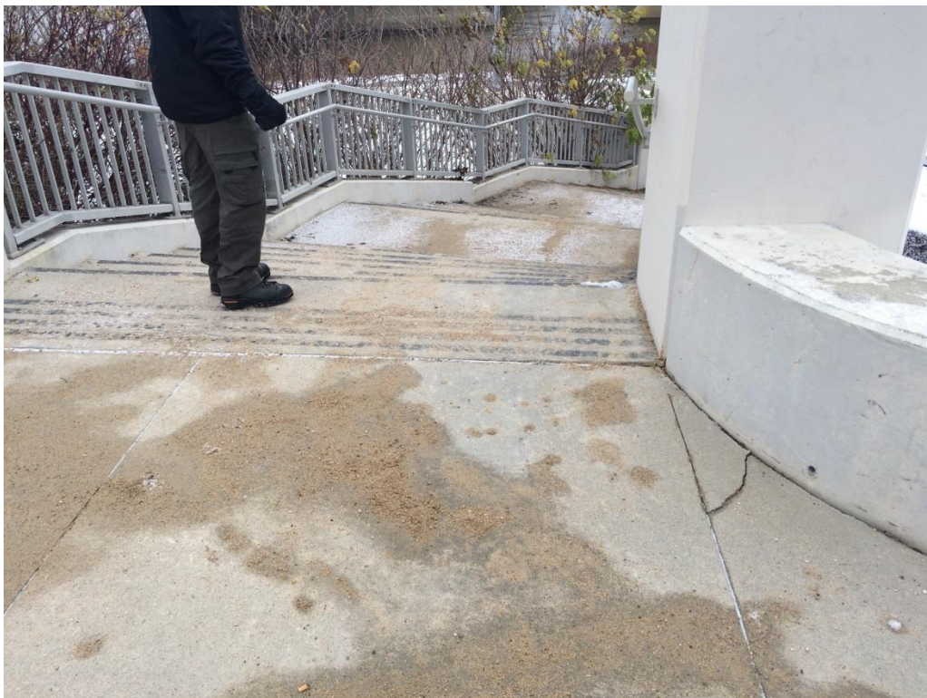
West Abutment Plaza - Location 4
