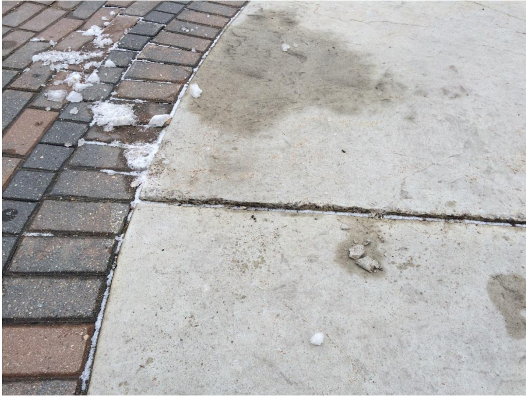
West Abutment Plaza - Location 3
