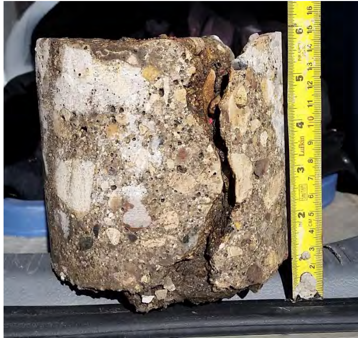
Figure 5: TH5– 150 mm cracked concrete
