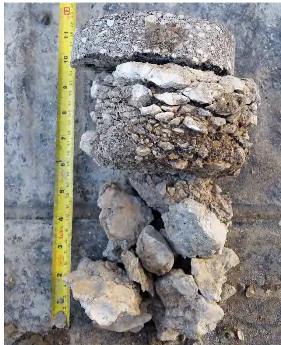
Figure 22: TH22 – 50 mm asphalt, 100 mm deteriorated concrete
