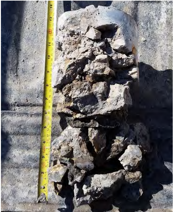
Figure 33: TH32 – 200 mm deteriorated concrete
