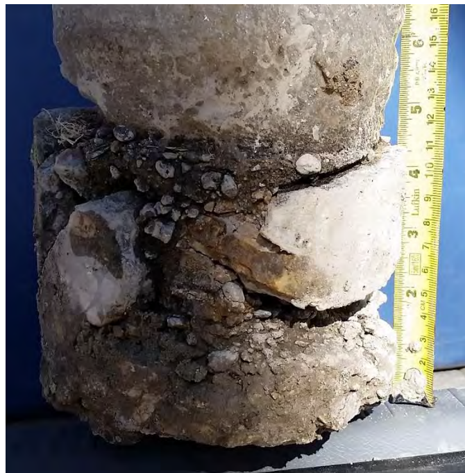
Figure 2: TH2 – 110 mm deteriorated concrete
