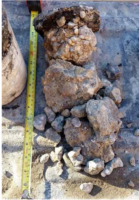
Figure 7: TH7 – 30 mm asphalt, 150 mm deteriorated concrete
