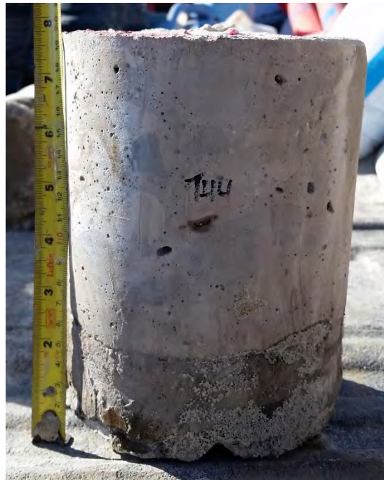
Figure 32: East end of alley, behind 360 Jefferson Ave – 200 mm intact concrete
