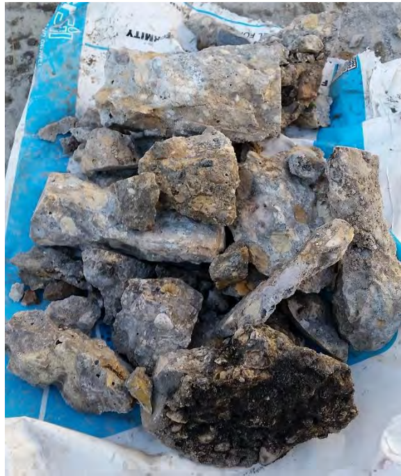
Figure 19: TH19 – 150 mm deteriorated concrete
