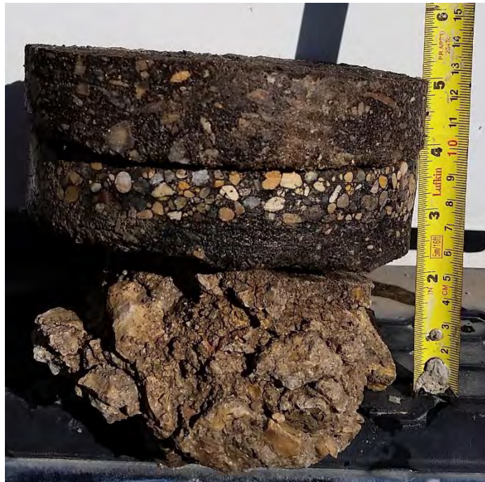
Figure 1: TH1 – 80 mm asphalt, 50 mm deteriorated concrete
