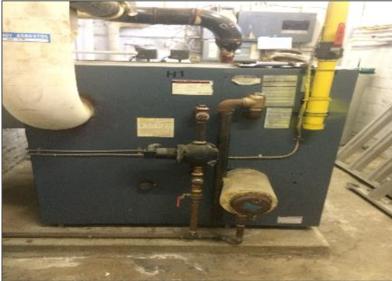
Photo #2: Refractory materials suspect to contain asbestos may be present beneath metal jacketing of boiler.
