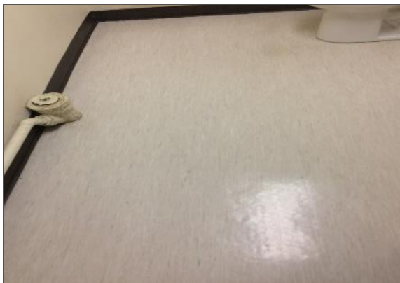
Photo #6: Non-asbestos vinyl sheet flooring with rubber backing within bathrooms.
