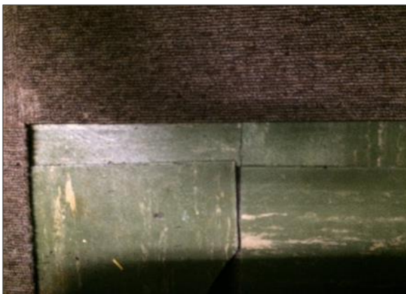
Photo #9: Asbestos-containing green floor tiles under carpet within the main floor library.
