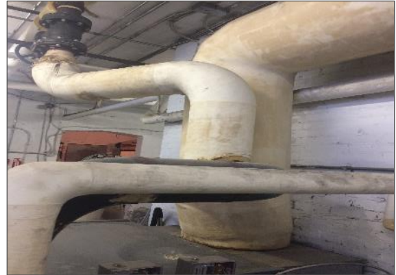
Photo #3: Non-asbestos fiberglass present on boiler breaching.
