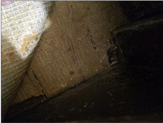
Photo #8: Non-asbestos battle ship flooring under carpeting within the basement corridor (Samples 0010).
