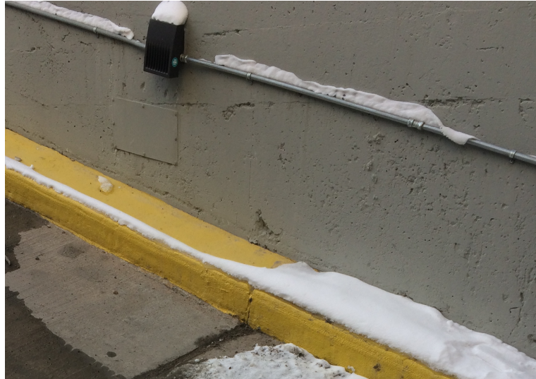
Figure 3 – Concrete along outer wall of Ramp 4.
