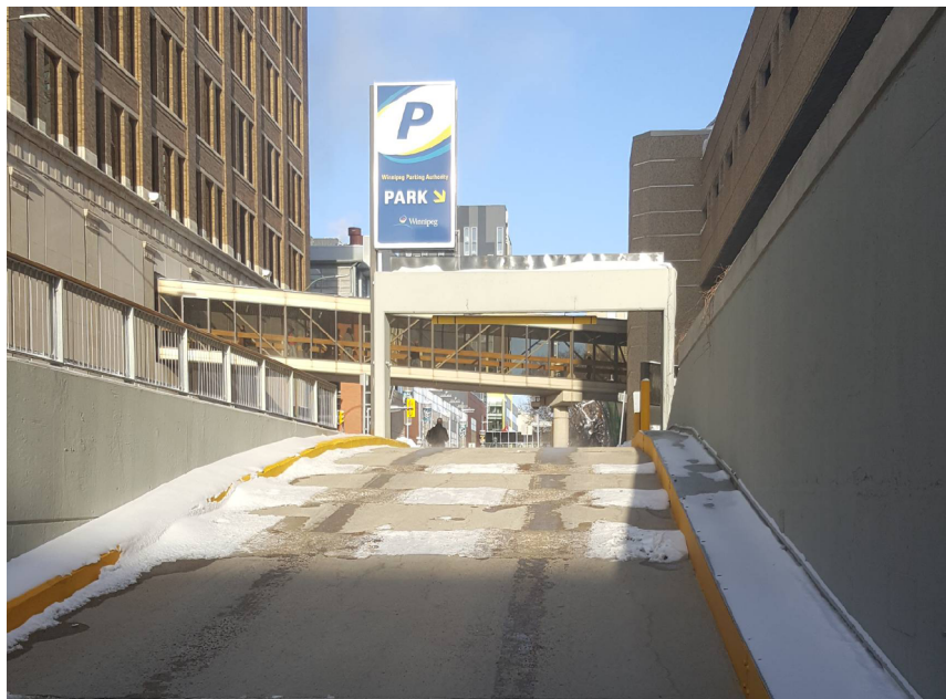
Figure 2 - Failed Sections of Donald street snow melt system
