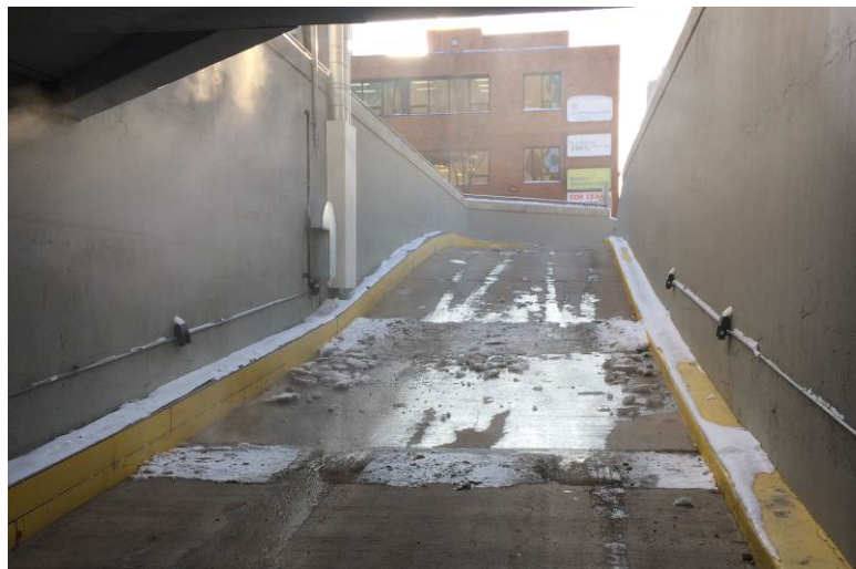
Figure 4 – Failed sections of Ramp 5 snow melt system
