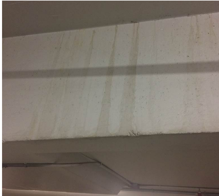
Figure 1 – Staining along interior wall beneath Ramp 2.
