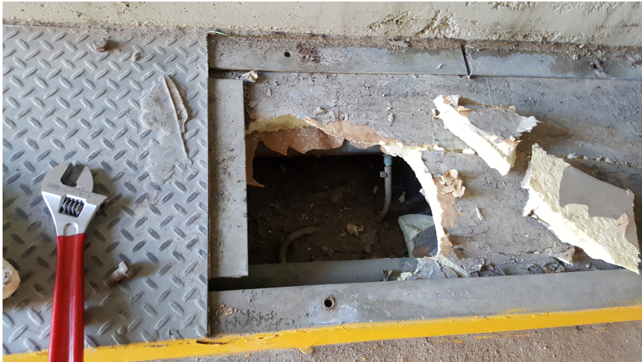
Figure 1 - Glycol distribution hoses from header
