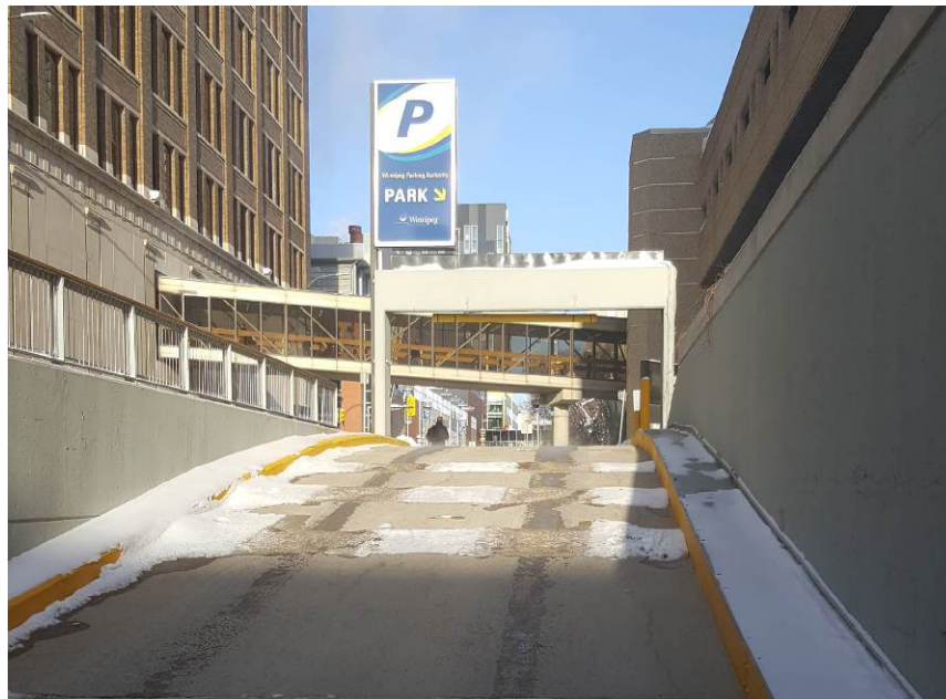
Figure 5 – Failed sections of Ramp 6 snow melt system.
