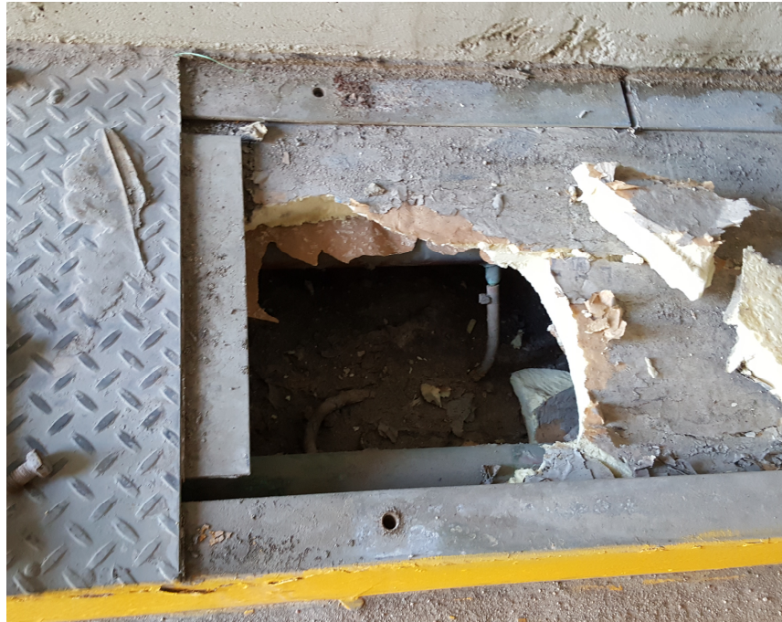
Figure 6 – Glycol distribution hoses from header in Ramp 6.
