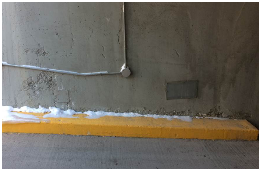
Figure 2 – Deteriorated concrete along outer wall of Ramp 3.
