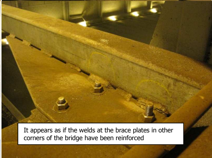
Evidence of prior repairs to SW corner of the bridge. Patch welds, on the members and stitch welds at the joint
