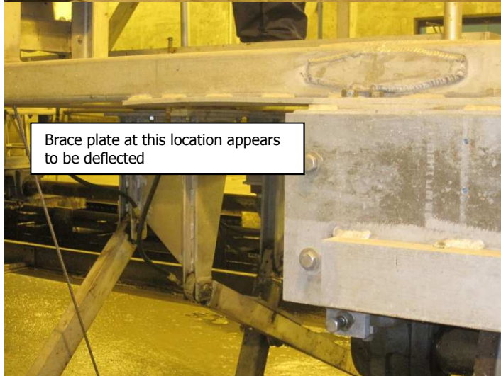
Evidence of prior repairs to SW corner of the bridge. Patch welds, on the members and stitch welds at the joint
