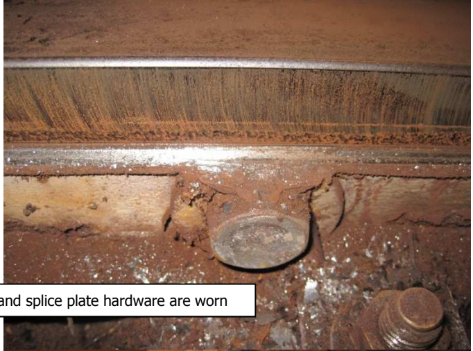
Head of rail worn flat, and signs of flaking, along entire length of rail
