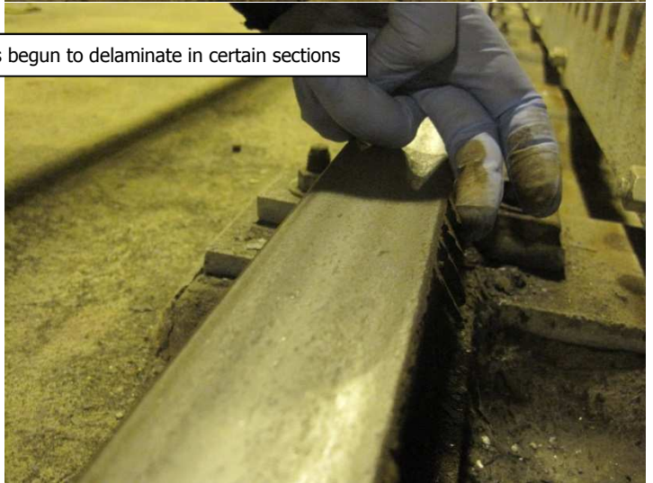
Head of rail worn flat along entire length, with pancaking in certain locations
