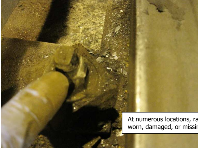
At most rail splices, top edge of splice plate itself, and splice plate hardware are worn
