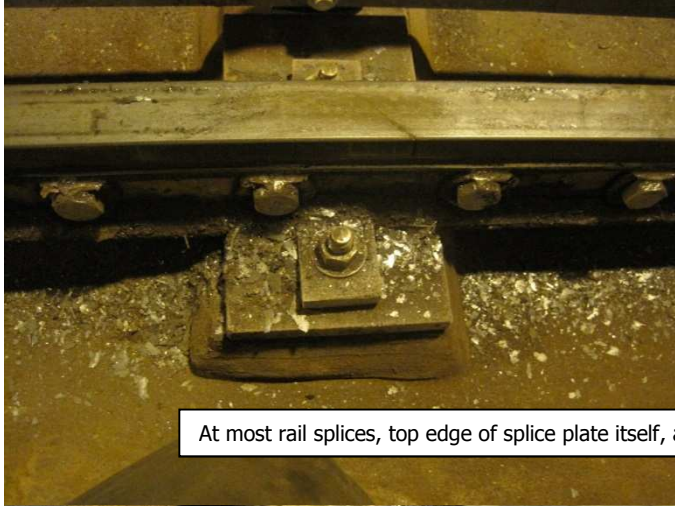
Head of rail worn flat, and signs of flaking, along entire length of rail
