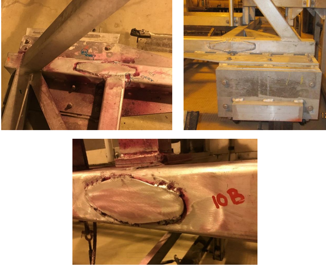
Figure 5: Field-Welded Plates
